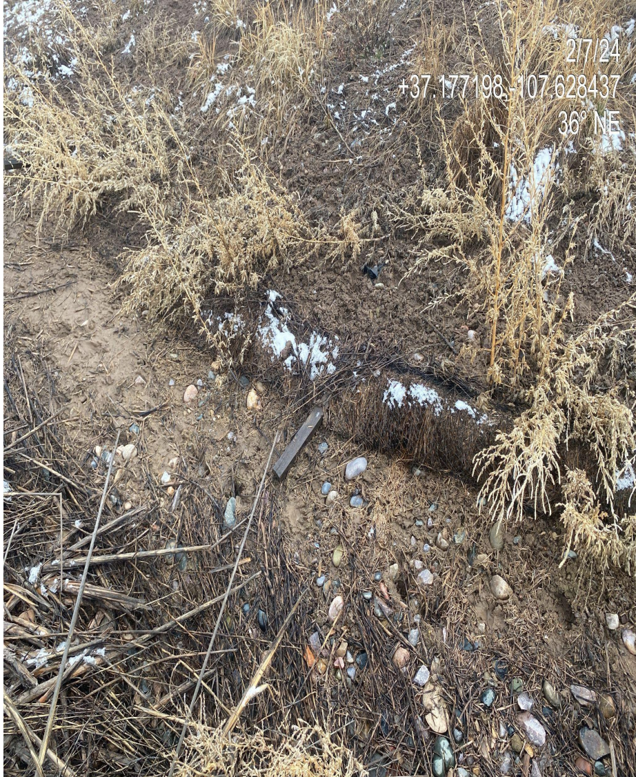
Photo 3. View of wattles no longer functioning at the base of the western cut slope and rill erosion forming up slope of the wattles.
