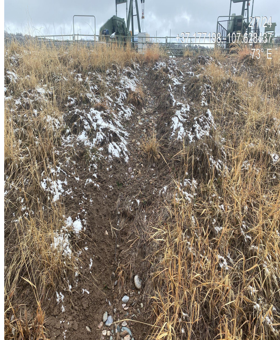
Photo 3. View of wattles no longer functioning at the base of the western cut slope and rill erosion forming up slope of the wattles.
