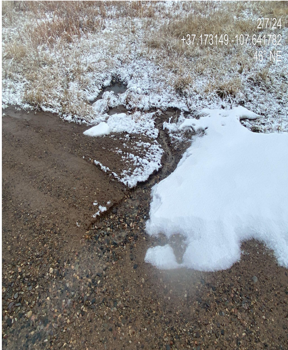
Photo 3. Rill erosion forming on the eastern edge of the disturbance near the access point.
