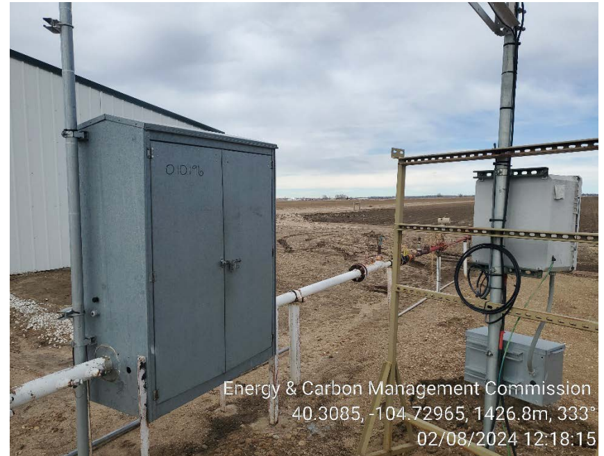
Meter run and automation array
