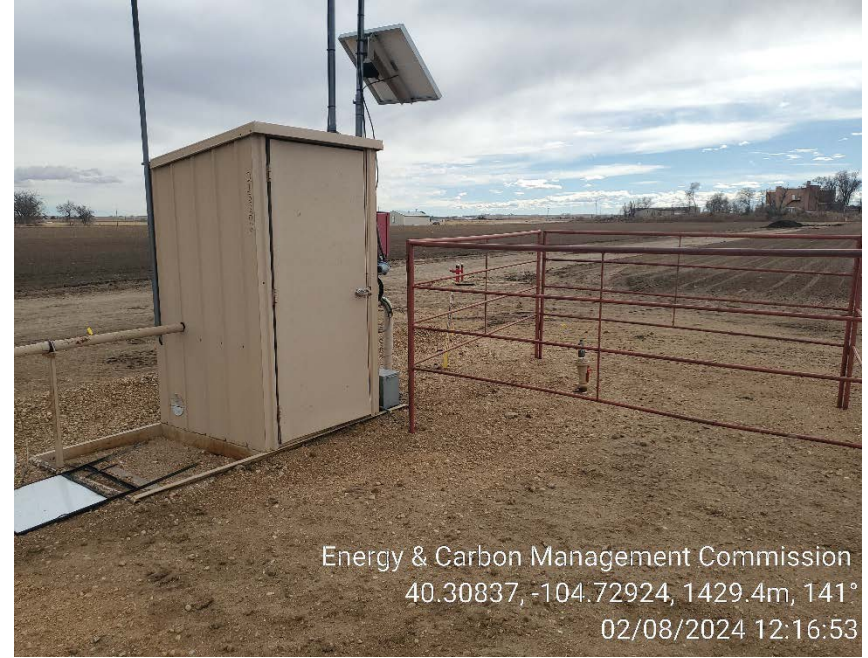
DCP meter run and flowline
