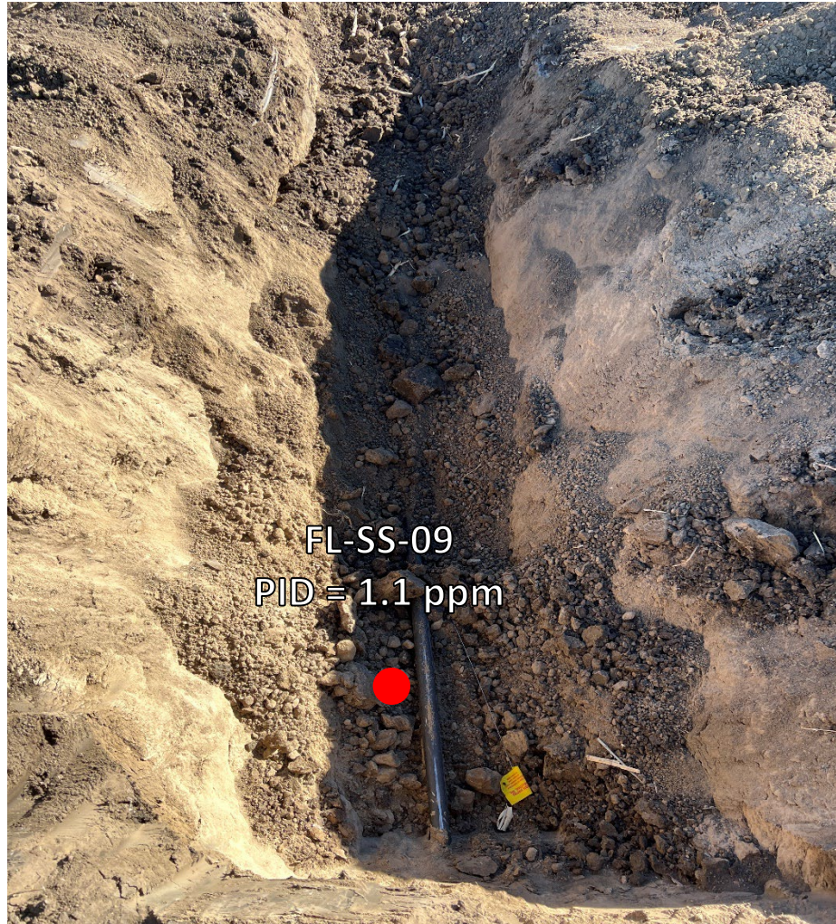
Looking east at bellhole/cut point for removal
