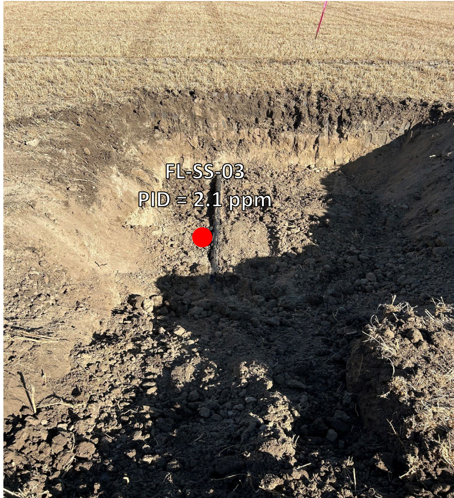
Looking north at flowline directional change
