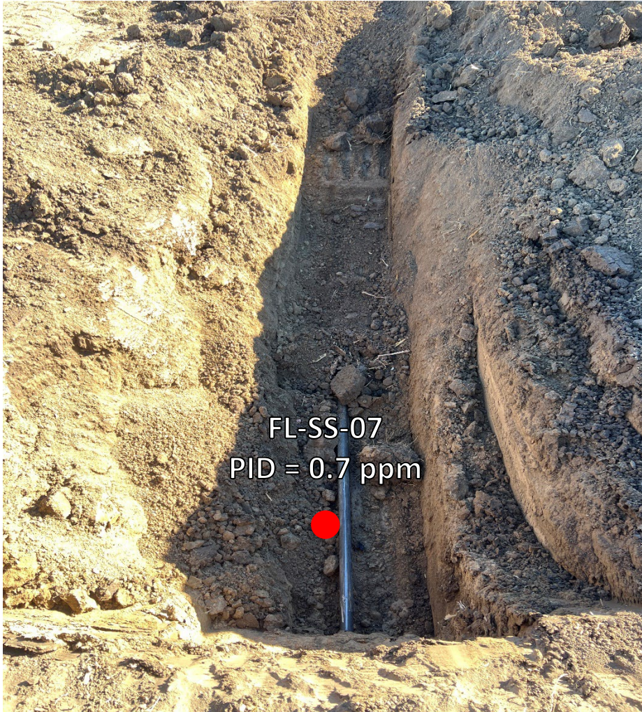
Looking east at bellhole/cut point for removal
