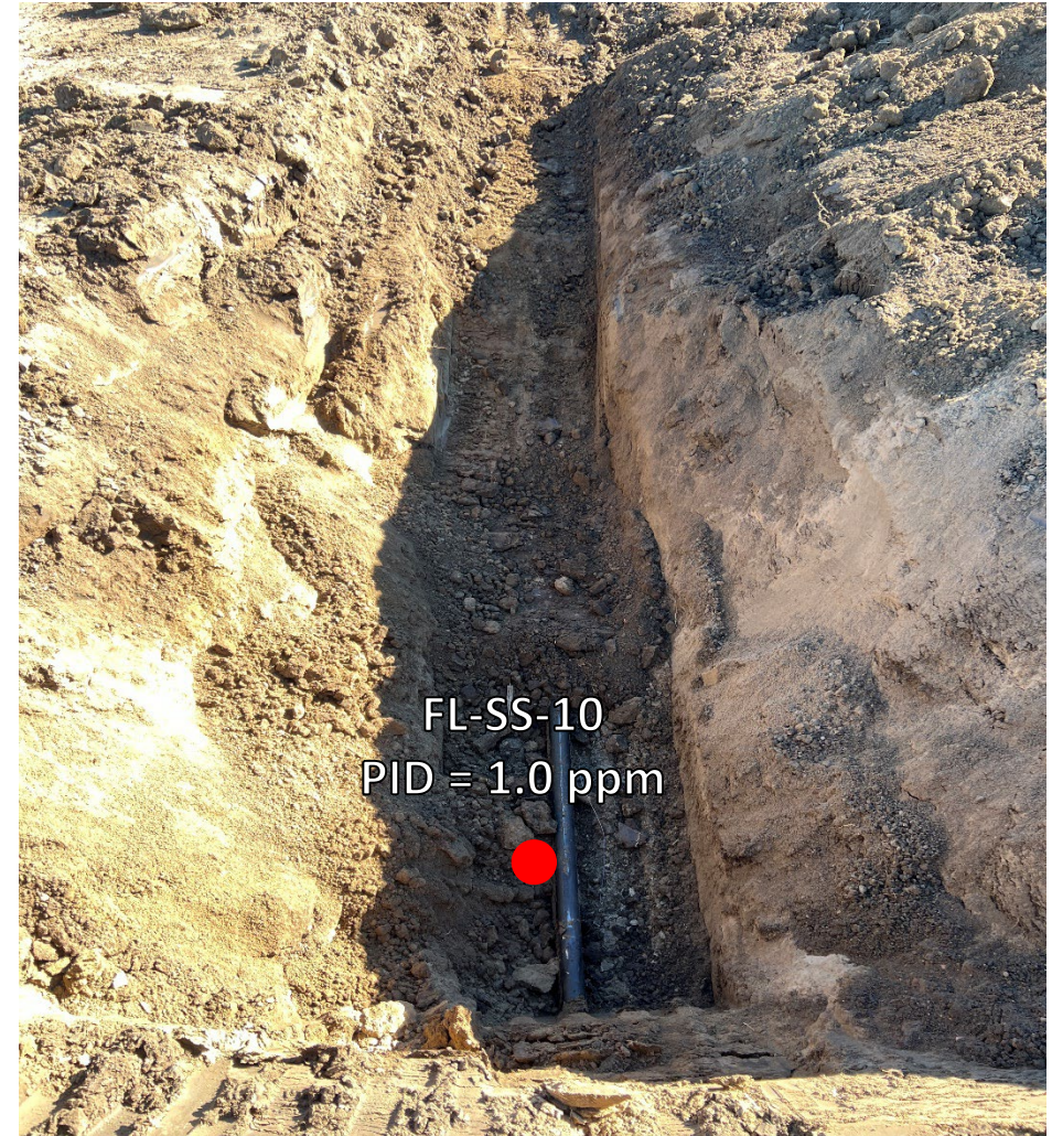
Looking east at bellhole/cut point for removal
