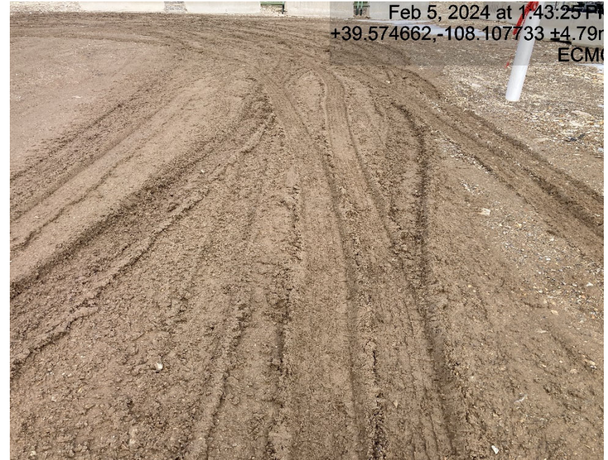
Lack of stabilization/compaction
