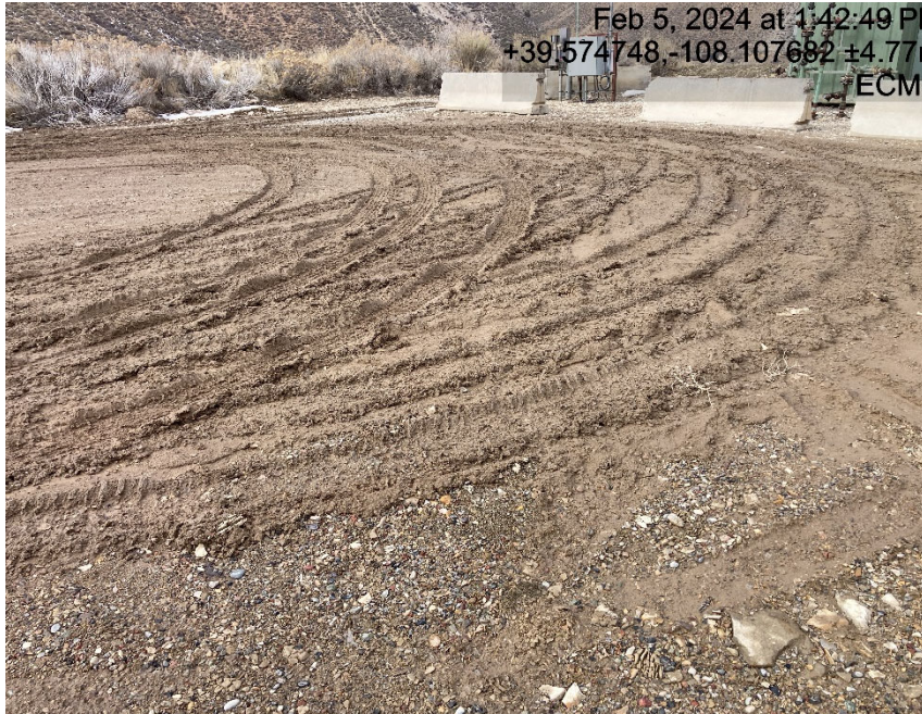
Lack of stabilization/compaction
