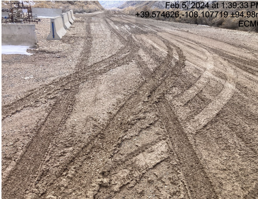
Lack of stabilization/compaction
