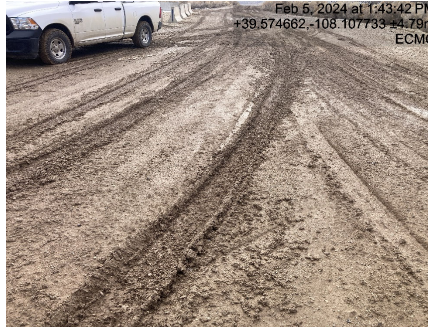
Lack of stabilization/compaction
