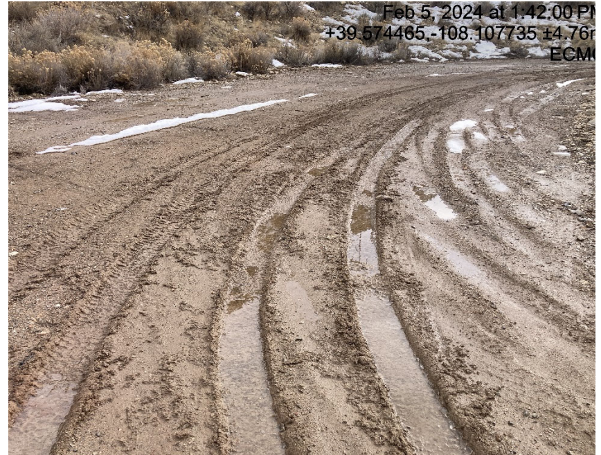
Lack of stabilization/compaction
