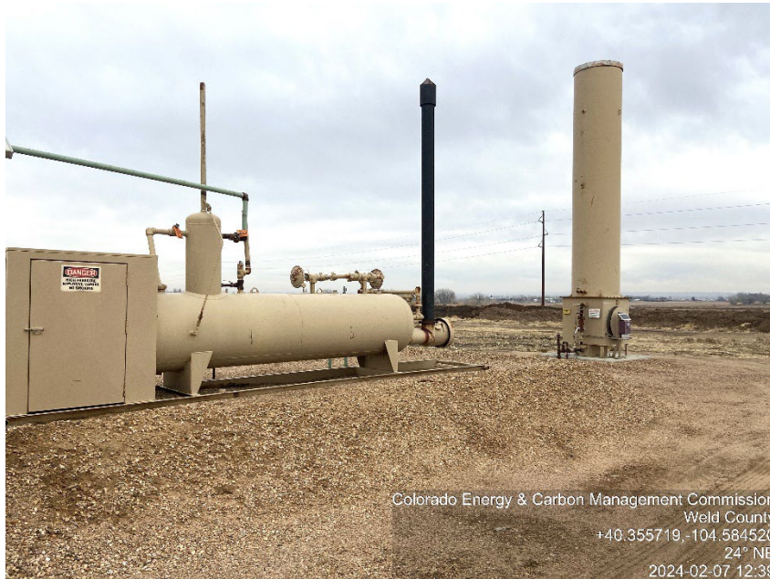
Photo #3 Thistle Down B 31-17 Battery site Inactive | Shut-down ECD(s), Separator(s)
