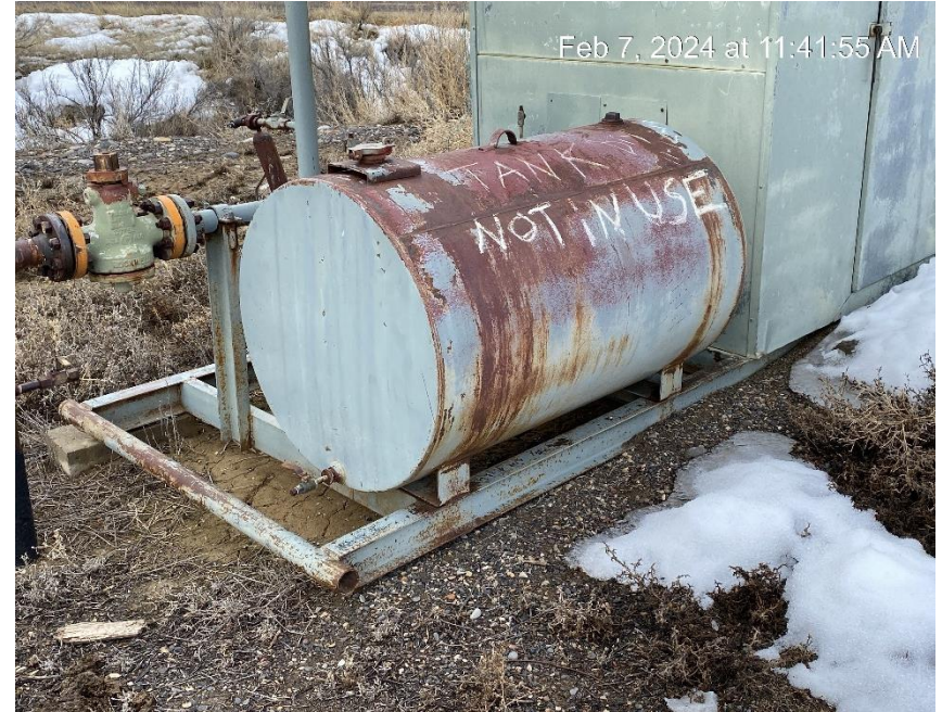
Accepted. Tank is welded to skid.
