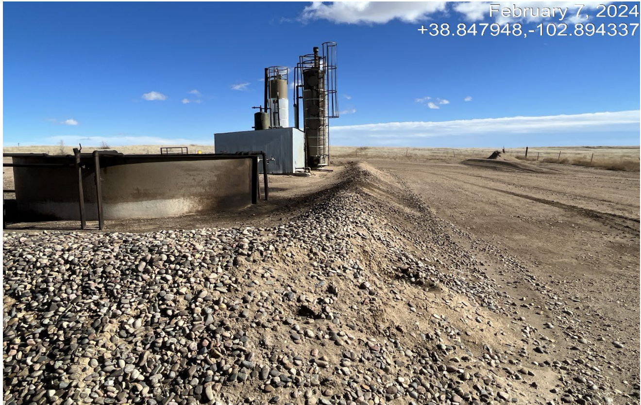
Photo 6. Facing east toward the backside of the open top tank. It appears some staining is along the outside of the berm.
