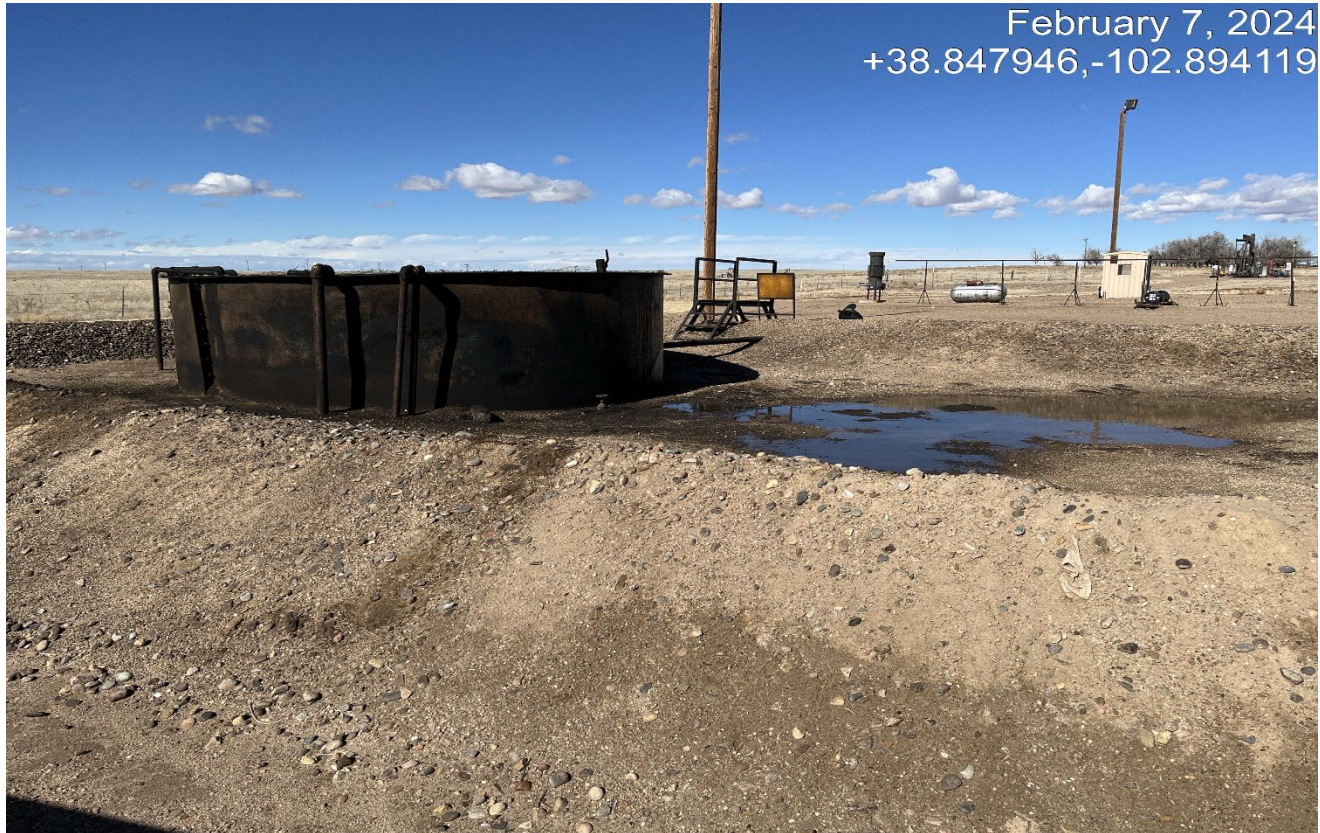
Photo 7. Facing toward the backside of the open top tank. Stained soils will need to be cleaned up..
