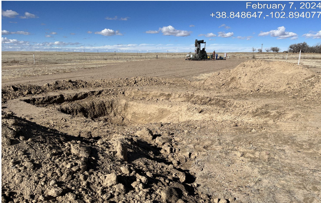
Photo 3. Facing northwest. There is an open excavation along the pipeline. This area should be marked with cones or safety fence to prevent accidental entry. .
