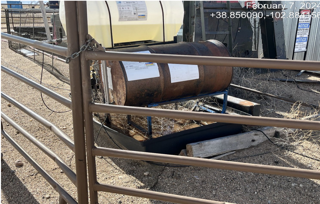
Photo 3. There is oily fluids inside the secondary containment of the barrels.
