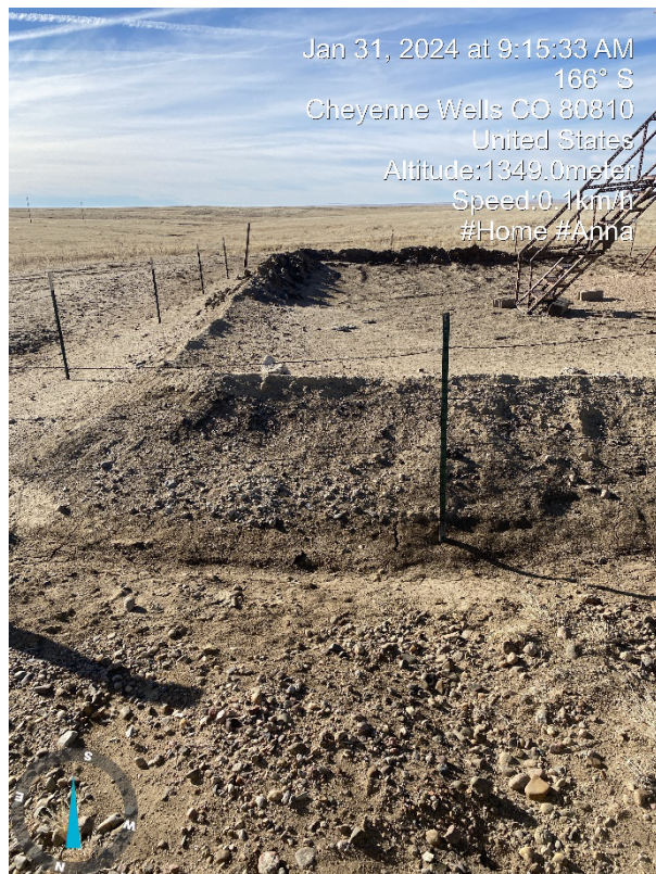
5. NE side of battery, Inadequate berms
