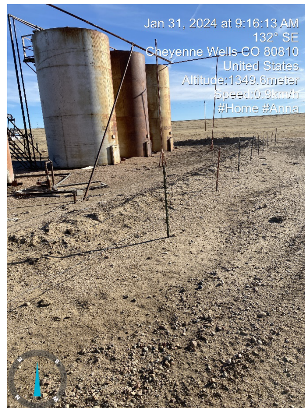
4. Back side of battery, Inadequate berms
