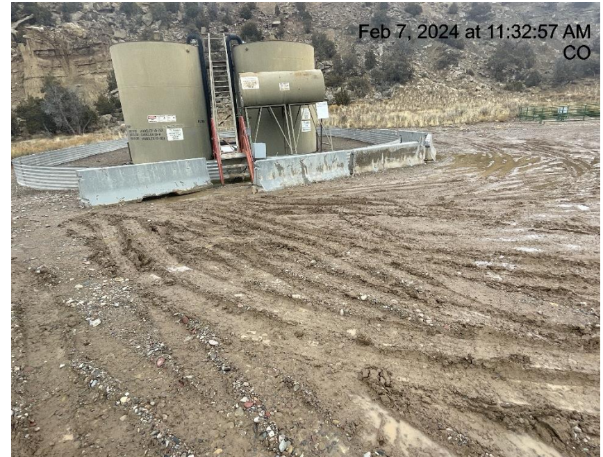
Photo # 5908 Lack of stabilization/compaction/insufficient tracking BMP's
