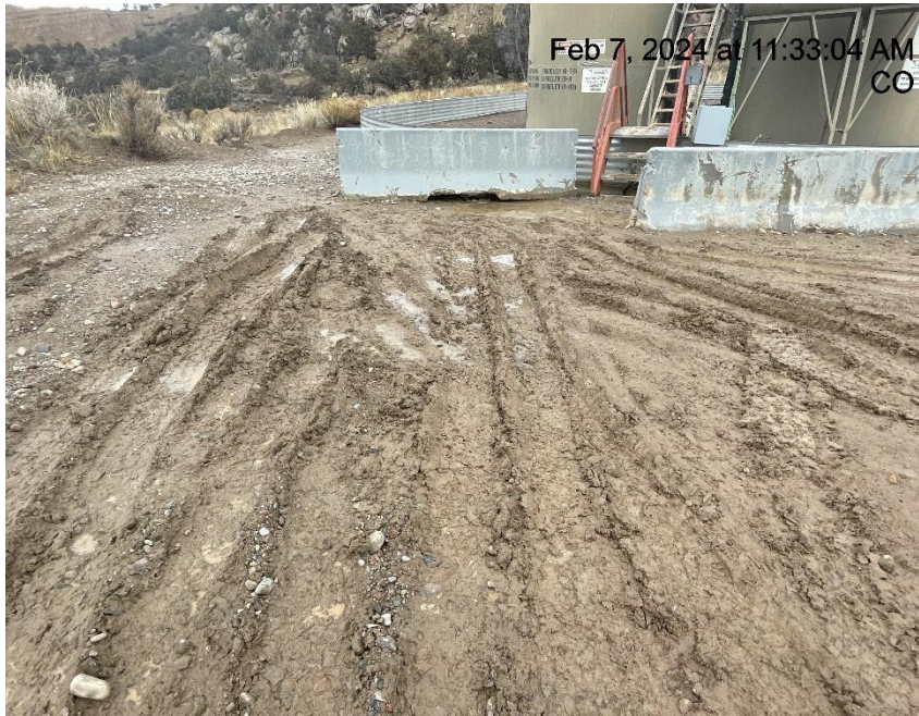
Photo # 5909 Lack of stabilization/compaction/insufficient tracking BMP's
