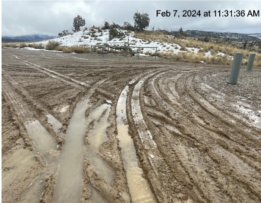
Photo # 5905 Lack of stabilization/compaction/insufficient tracking BMP's
