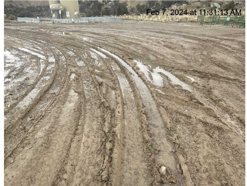
Photo # 5902 Lack of stabilization/compaction/insufficient tracking BMP's
