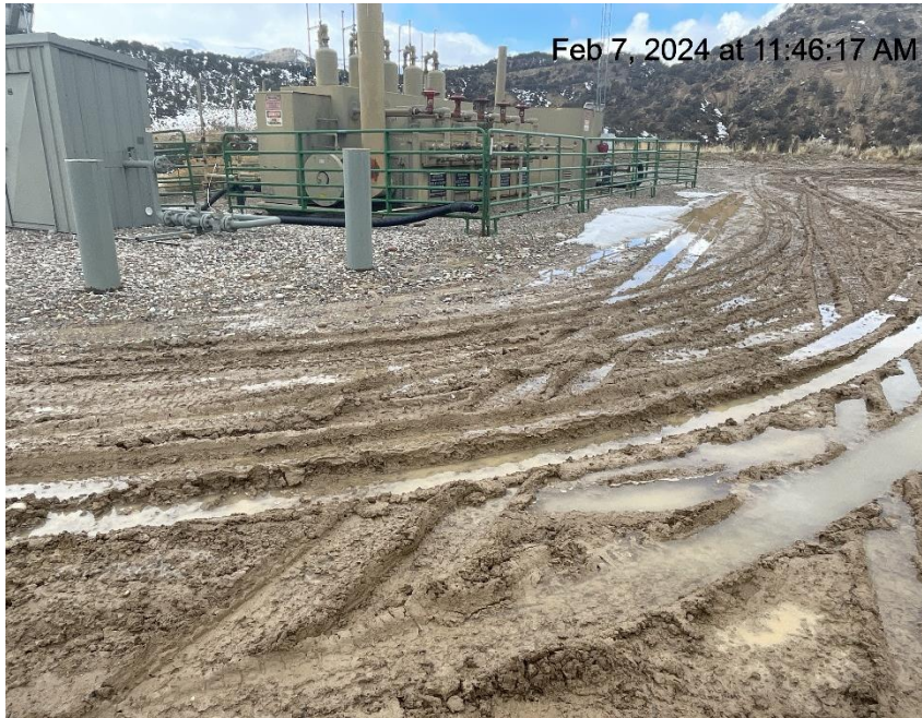
Photo # 5907 Lack of stabilization/compaction/insufficient tracking BMP's
