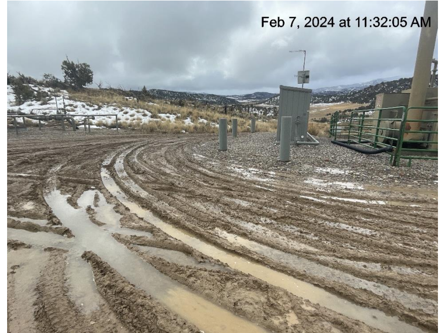
Photo # 5906 Lack of stabilization/compaction/insufficient tracking BMP's
