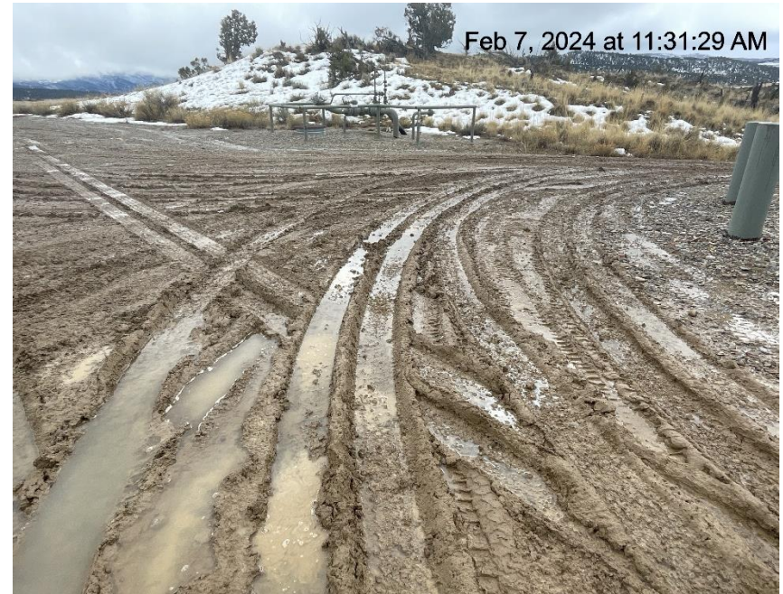
Photo # 5904 Lack of stabilization/compaction/insufficient tracking BMP's
