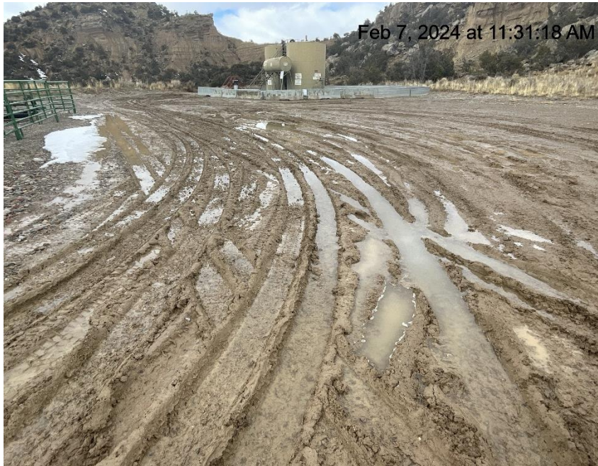
Photo # 5903 Lack of stabilization/compaction/insufficient tracking BMP's
