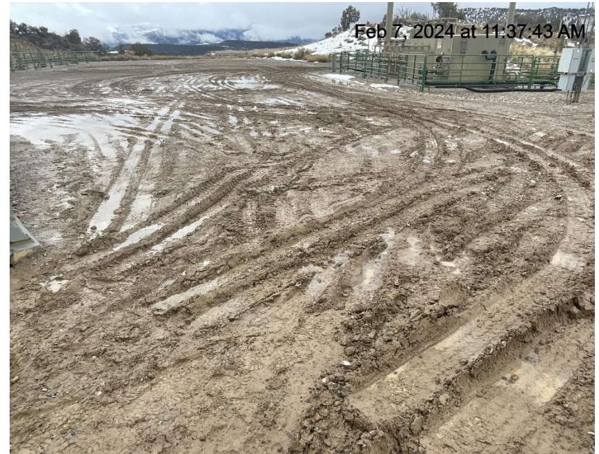
Photo # 5910 Lack of stabilization/compaction/insufficient tracking BMP's
