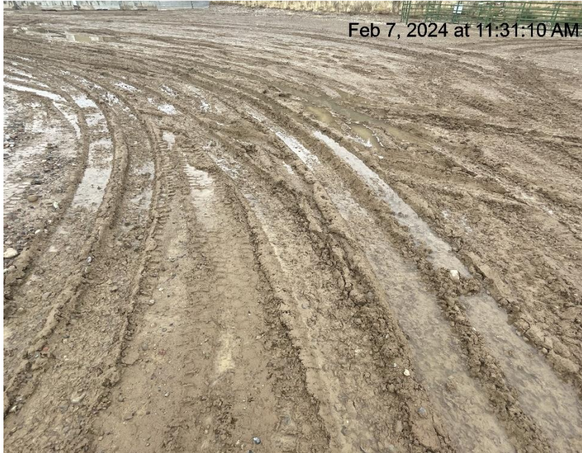
Photo # 5901 Lack of stabilization/compaction/insufficient tracking BMP's
