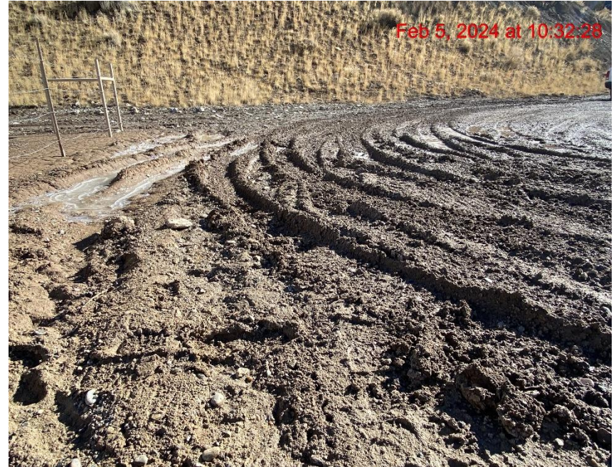
Lack of Stabilization – Photo #09117
