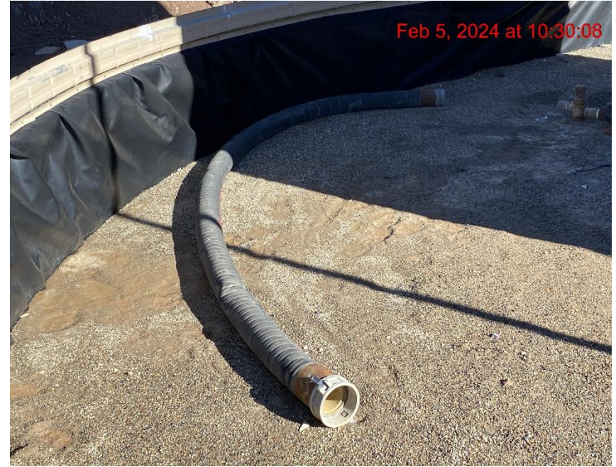
Stored Equipment – Photo #09111
