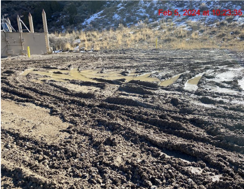
Lack of Stabilization – Photo #09105
