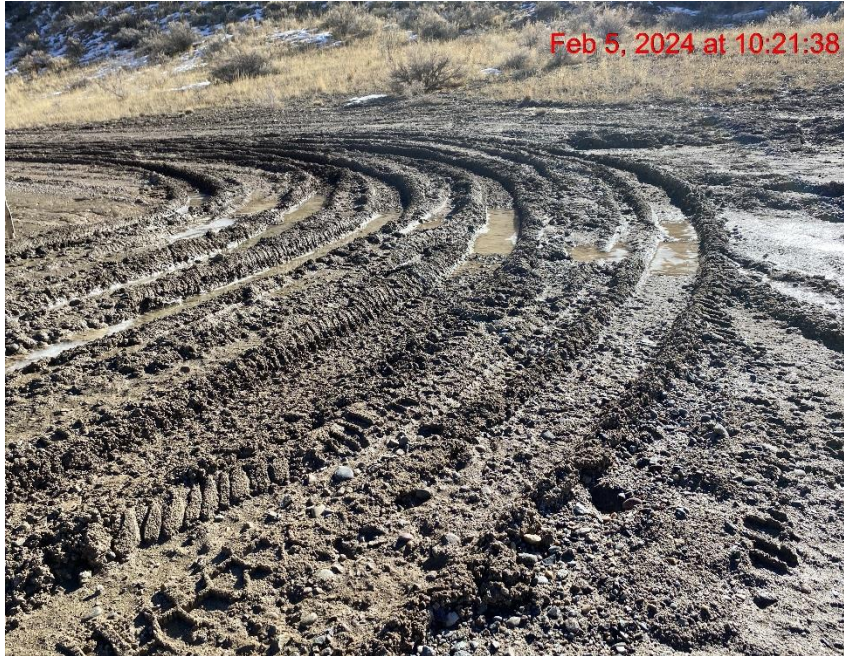
Lack of Stabilization – Photo #09102
