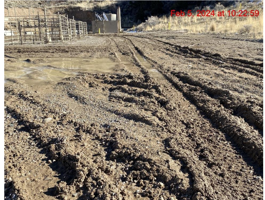
Lack of Stabilization – Photo #09104
