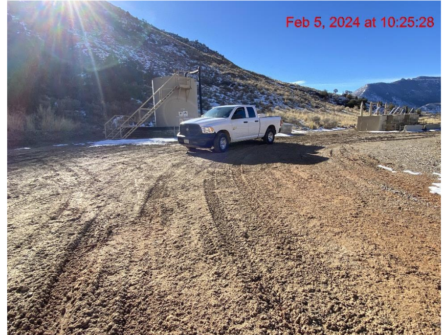
Insufficient Vehicle Tracking BMPs at Location Entrance/Exit – Photo #09106
