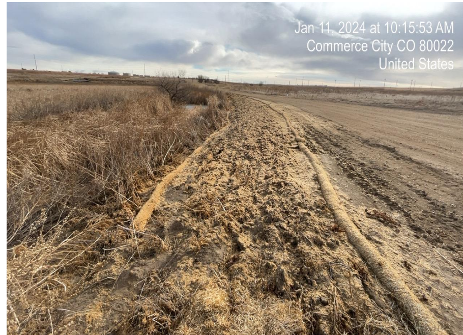
Photo 6. Photo taken of reseeded area along access road and wattles. Photo taken facing southeast.
