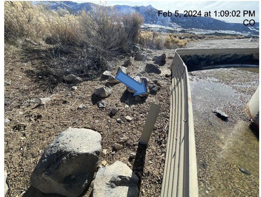
Photo # 5778 Tank battery containment starting to buckle & has separated from one of the support braces.
