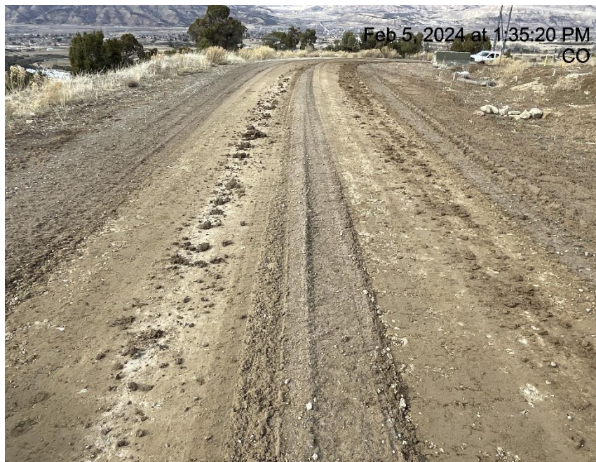
Photo # 5737 Insufficient tracking BMP's at entrance to location/tracking onto lease road
