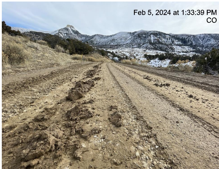
Photo # 5731 Insufficient tracking BMP's at entrance to location/tracking onto lease road
