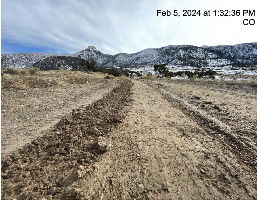
Photo # 5725 Insufficient tracking BMP's at entrance to location/tracking onto lease road
