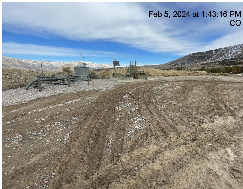
Photo # 5745 Lack of stabilization/compaction/insufficient tracking BMP's
