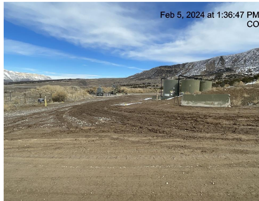
Photo # 5716 Lack of stabilization/compaction/insufficient tracking BMP's at entrance to location/tracking onto lease road
