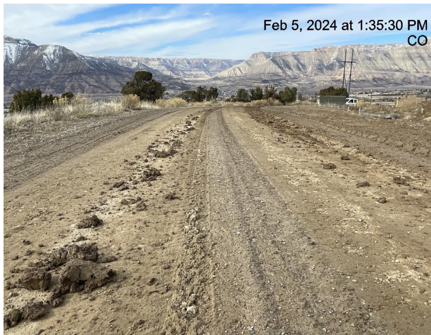
Photo # 5739 Insufficient tracking BMP's at entrance to location/tracking onto lease road
