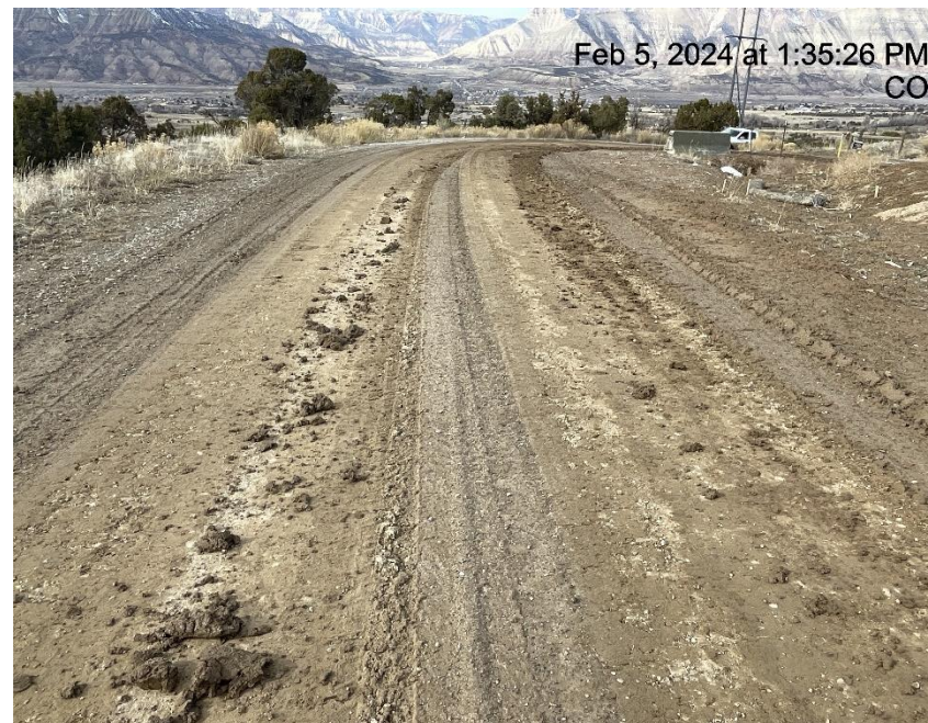
Photo # 5738 Insufficient tracking BMP's at entrance to location/tracking onto lease road
