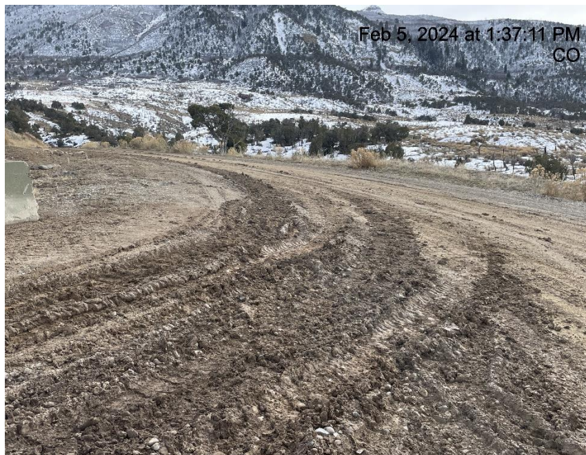
Photo # 5741 Insufficient tracking BMP's at entrance to location/tracking onto lease road
