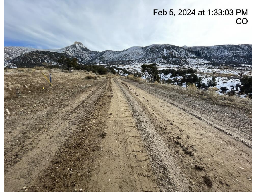
Photo # 5726 Insufficient tracking BMP's at entrance to location/tracking onto lease road
