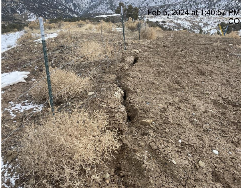
Photo # 5751 Soil starting to slough near fencing
