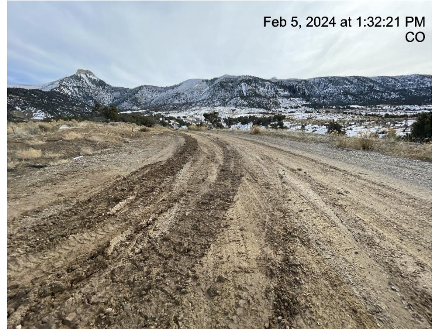
Photo # 5722 Insufficient tracking BMP's at entrance to location/tracking onto lease road
