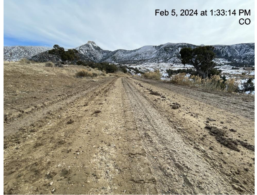
Photo # 5728 Insufficient tracking BMP's at entrance to location/tracking onto lease road
