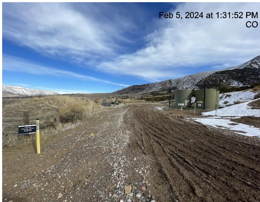
Photo # 5705 Lack of stabilization/compaction/insufficient tracking BMP's at entrance to location
