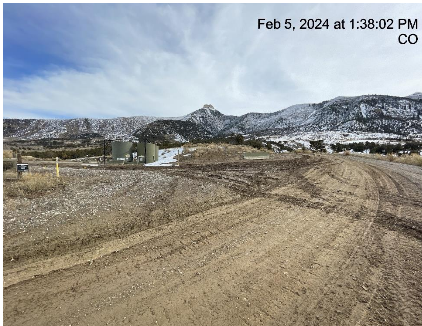
Photo # 5715 Lack of stabilization/compaction/insufficient tracking BMP's at entrance to location/tracking onto lease road
