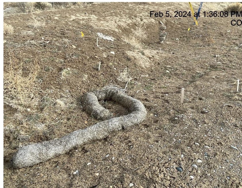
Photo # 5748 Wattle needs maintenance (on lease road near entrance to location)
