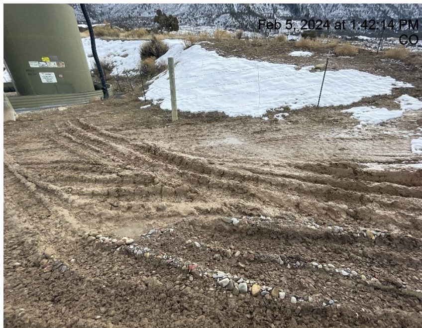
Photo # 5747 Lack of stabilization/compaction/insufficient tracking BMP's
