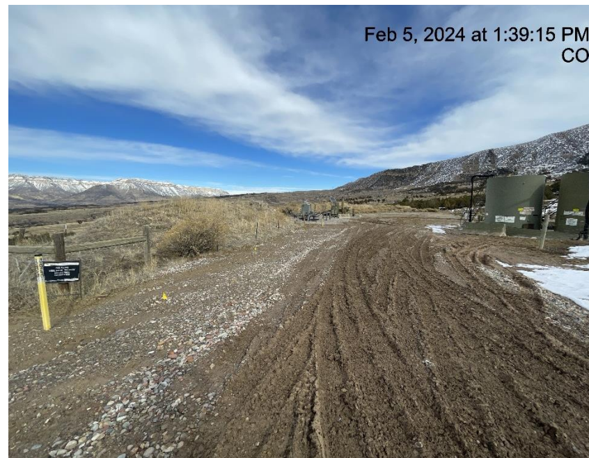
Photo # 5708 Lack of stabilization/compaction/insufficient tracking BMP's at entrance to location
