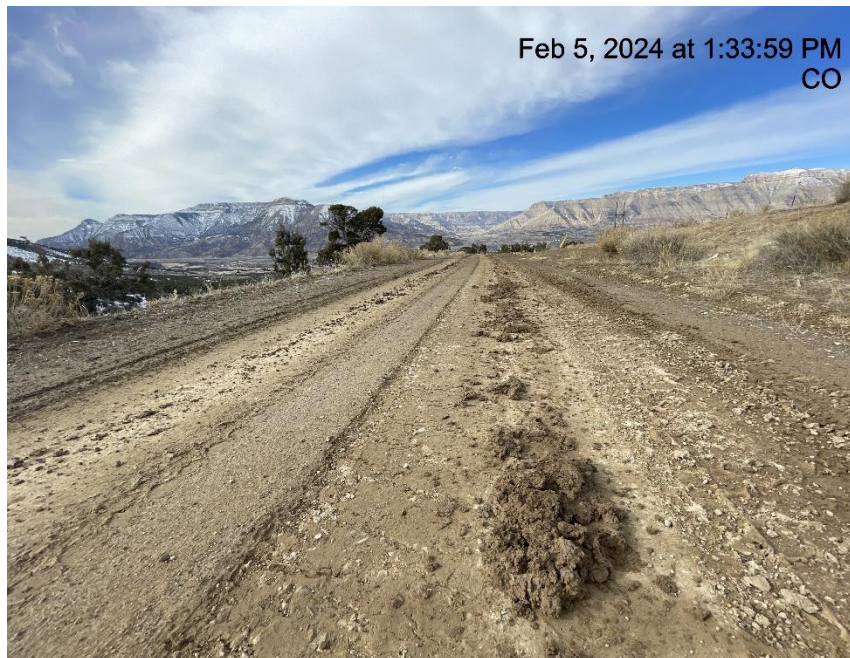
Photo # 5733 Insufficient tracking BMP's at entrance to location/tracking onto lease road
