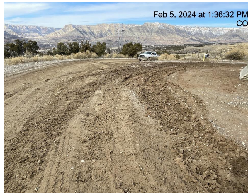
Photo # 5740 Insufficient tracking BMP's at entrance to location/tracking onto lease road
