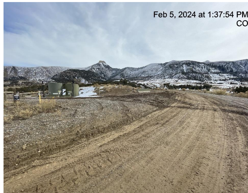
Photo # 5742 Insufficient tracking BMP's at entrance to location/tracking onto lease road
