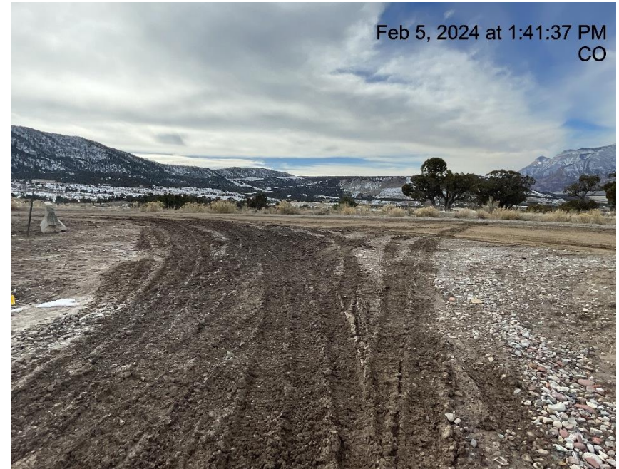
Photo # 5710 Lack of stabilization/compaction/insufficient tracking BMP's at entrance to location
