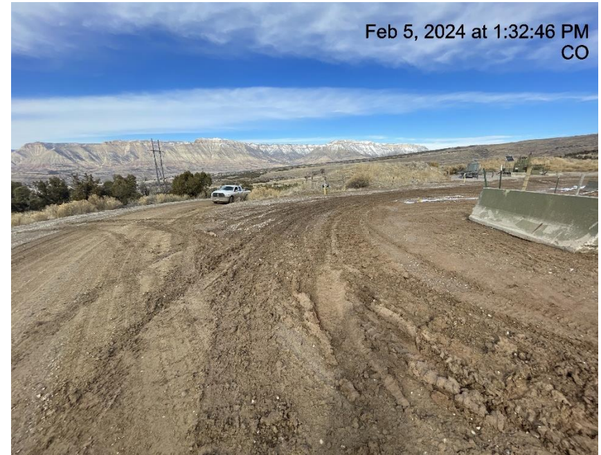
Photo # 5720 Insufficient tracking BMP's at entrance to location/tracking onto lease road
