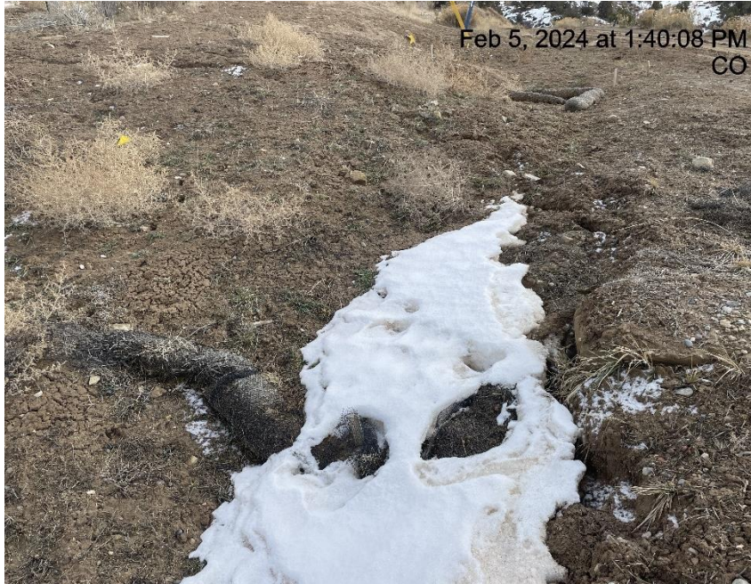
Photo # 5749 Wattle needs maintenance (on lease road near entrance to location)
