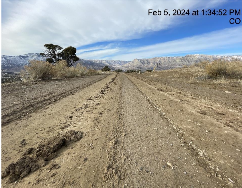
Photo # 5735 Insufficient tracking BMP's at entrance to location/tracking onto lease road
