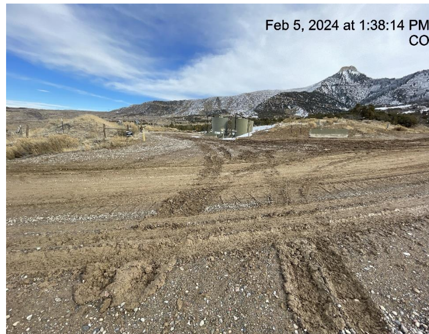
Photo # 5714 Lack of stabilization/compaction/insufficient tracking BMP's at entrance to location/tracking onto lease road
