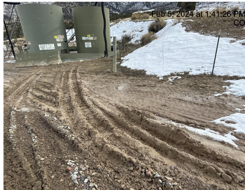
Photo # 5744 Lack of stabilization/compaction/insufficient tracking BMP's
