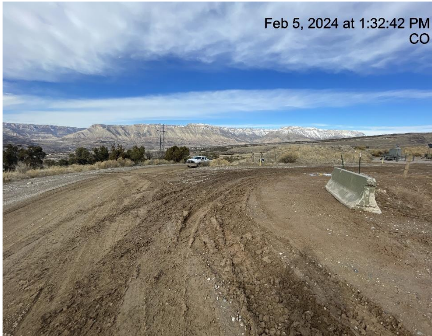
Photo # 5719 Insufficient tracking BMP's at entrance to location/tracking onto lease road
