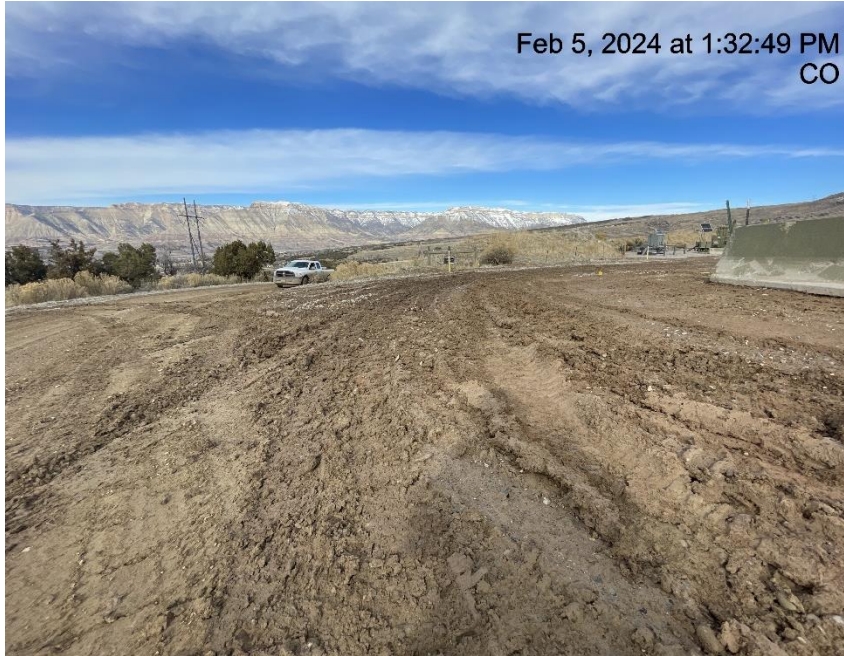
Photo # 5721 Insufficient tracking BMP's at entrance to location/tracking onto lease road
