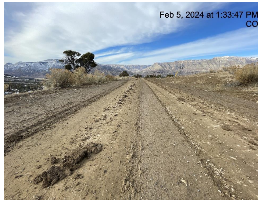
Photo # 5732 Insufficient tracking BMP's at entrance to location/tracking onto lease road
