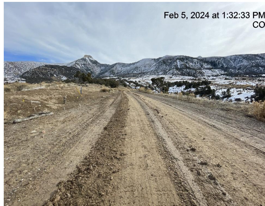
Photo # 5724 Insufficient tracking BMP's at entrance to location/tracking onto lease road
