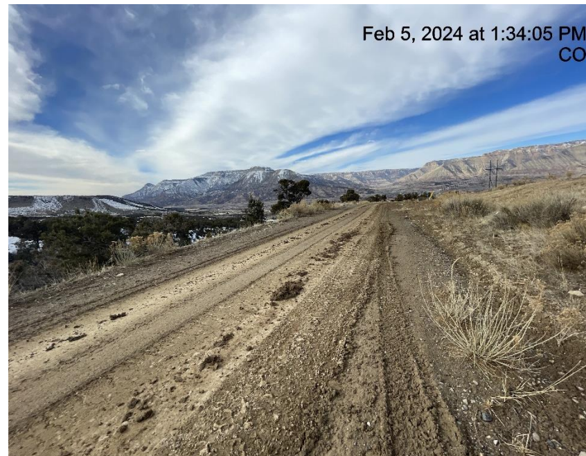
Photo # 5734 Insufficient tracking BMP's at entrance to location/tracking onto lease road
