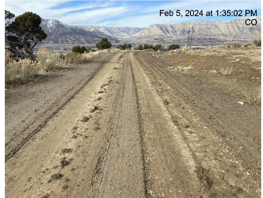
Photo # 5736 Insufficient tracking BMP's at entrance to location/tracking onto lease road
