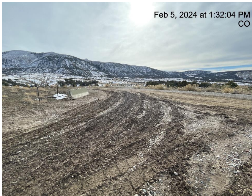
Photo # 5711 Lack of stabilization/compaction/insufficient tracking BMP's at entrance to location/tracking onto lease road
