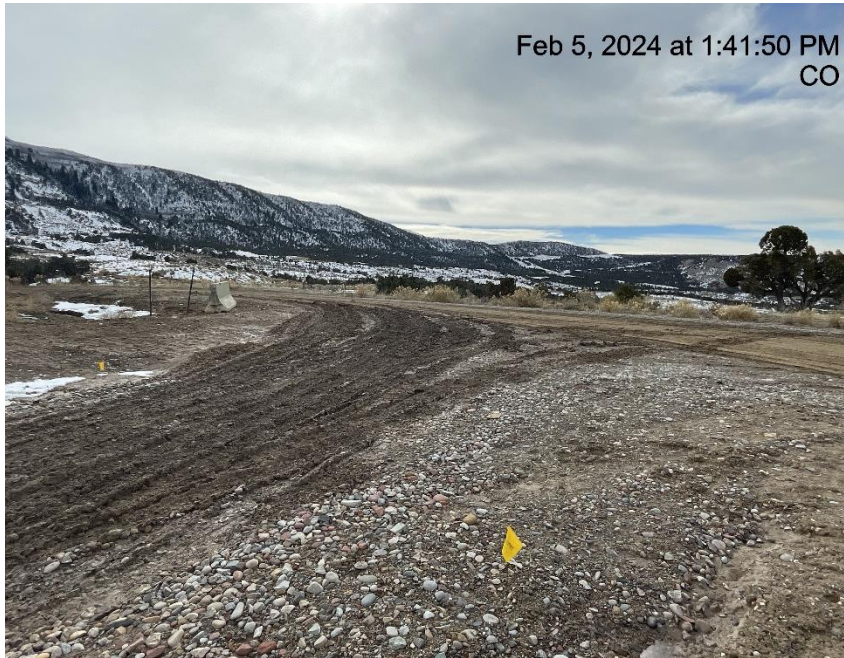
Photo # 5709 Lack of stabilization/compaction/insufficient tracking BMP's at entrance to location
