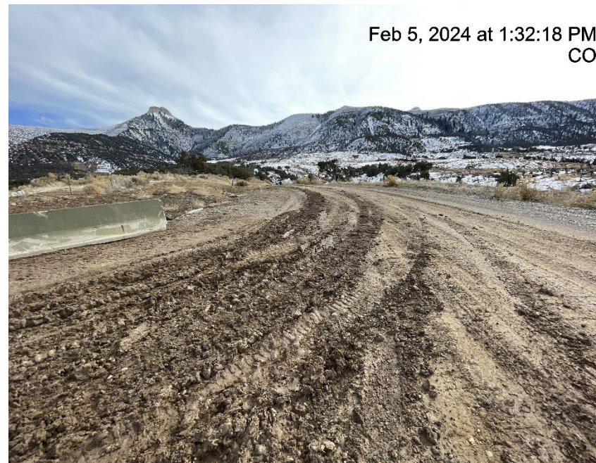
Photo # 5718 Insufficient tracking BMP's at entrance to location/tracking onto lease road
