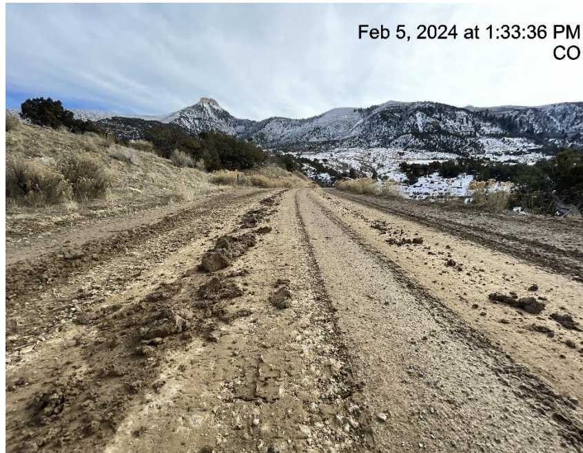
Photo # 5730 Insufficient tracking BMP's at entrance to location/tracking onto lease road
