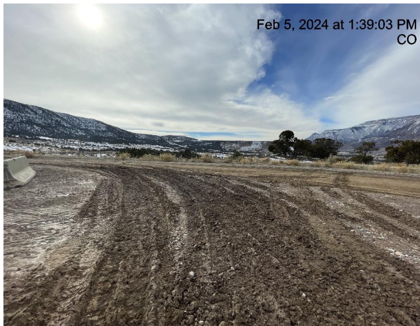
Photo # 5713 Lack of stabilization/compaction/insufficient tracking BMP's at entrance to location/tracking onto lease road
