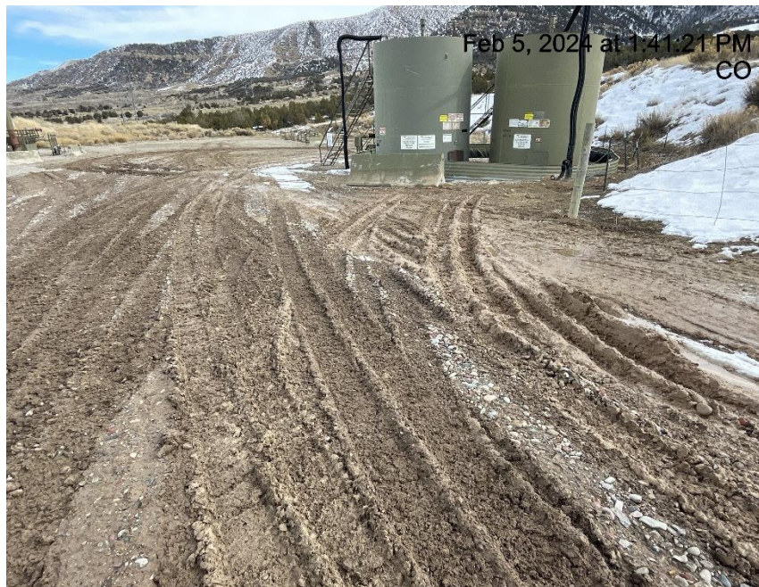
Photo # 5743 Lack of stabilization/compaction/insufficient tracking BMP's
