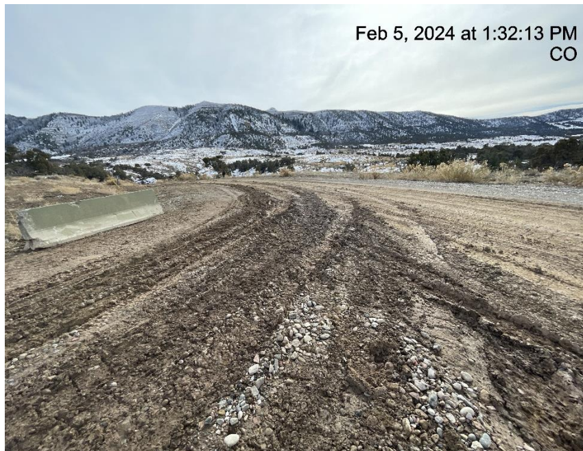
Photo # 5717 Insufficient tracking BMP's at entrance to location/tracking onto lease road
