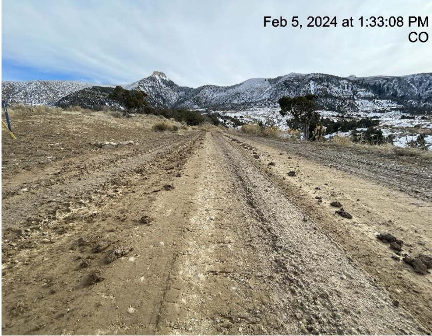
Photo # 5727 Insufficient tracking BMP's at entrance to location/tracking onto lease road
