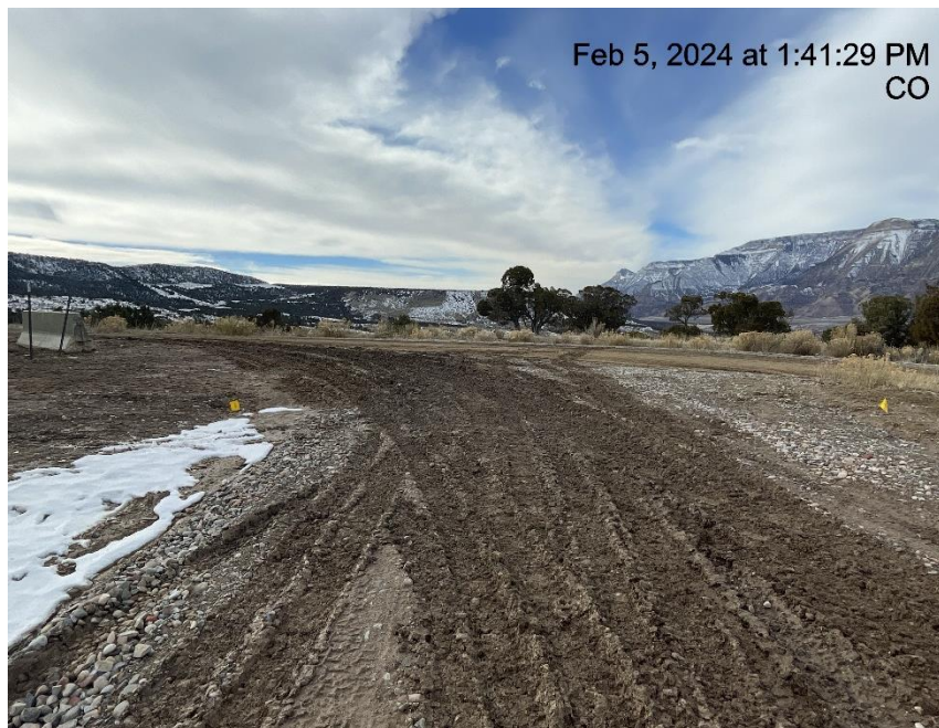
Photo # 5707 Lack of stabilization/compaction/insufficient tracking BMP's at entrance to location
