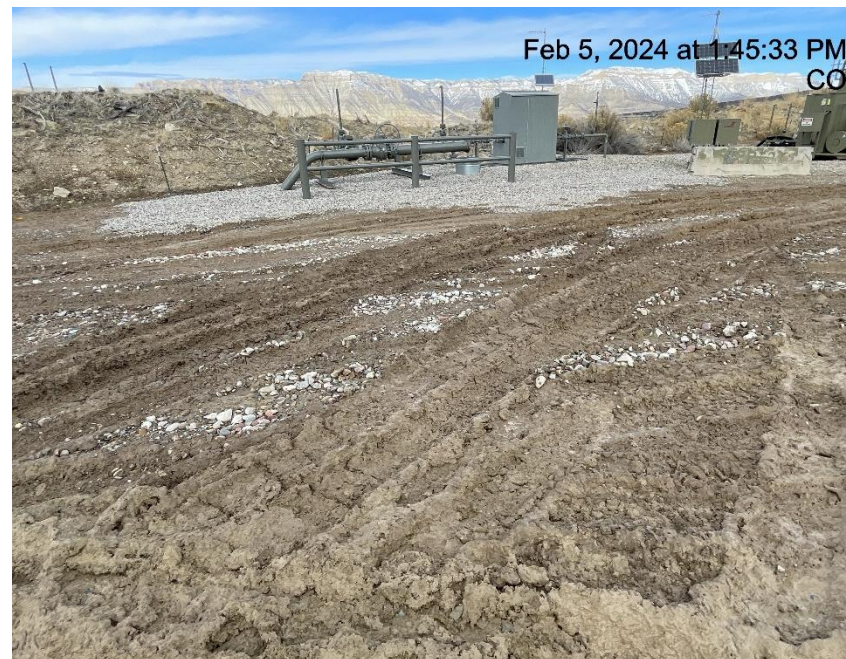
Photo # 5746 Lack of stabilization/compaction/insufficient tracking BMP's
