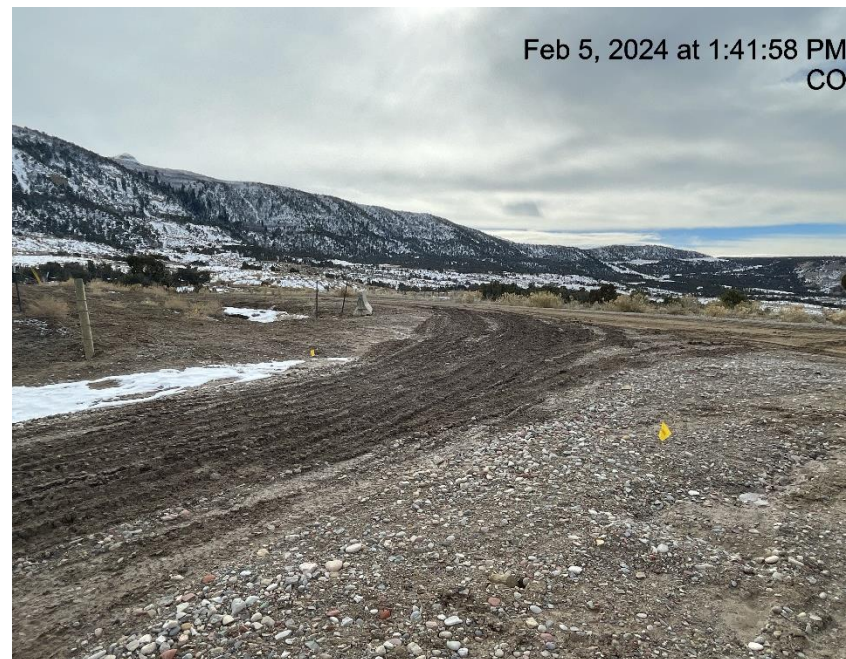
Photo # 5706 Lack of stabilization/compaction/insufficient tracking BMP's at entrance to location
