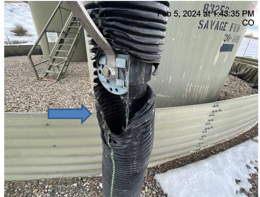
Photo # 5700 Hole in flowline heating insulation/wildlife hazard/available for entry by wildlife
