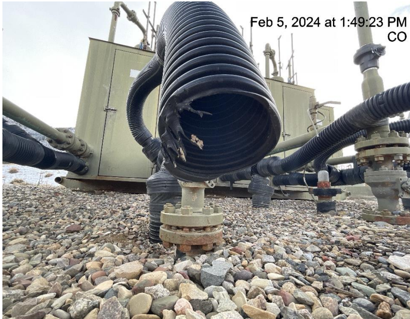
Photo # 5701 Flowline heating insulation open ended/wildlife hazard/available for entry by wildlife
