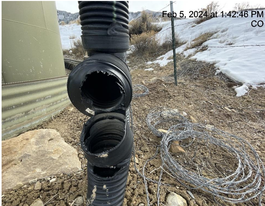
Photo # 5699 Flowline heating insulation open ended/wildlife hazard/available for entry by wildlife
