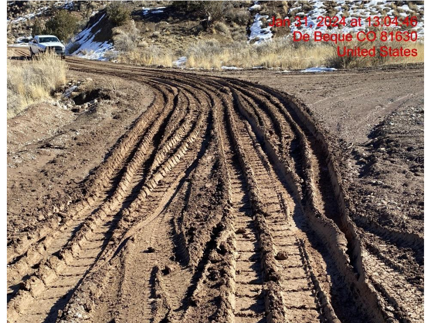
Insufficient Vehicle Tracking BMPs at Location Entrance/Exit – Photo #09049
