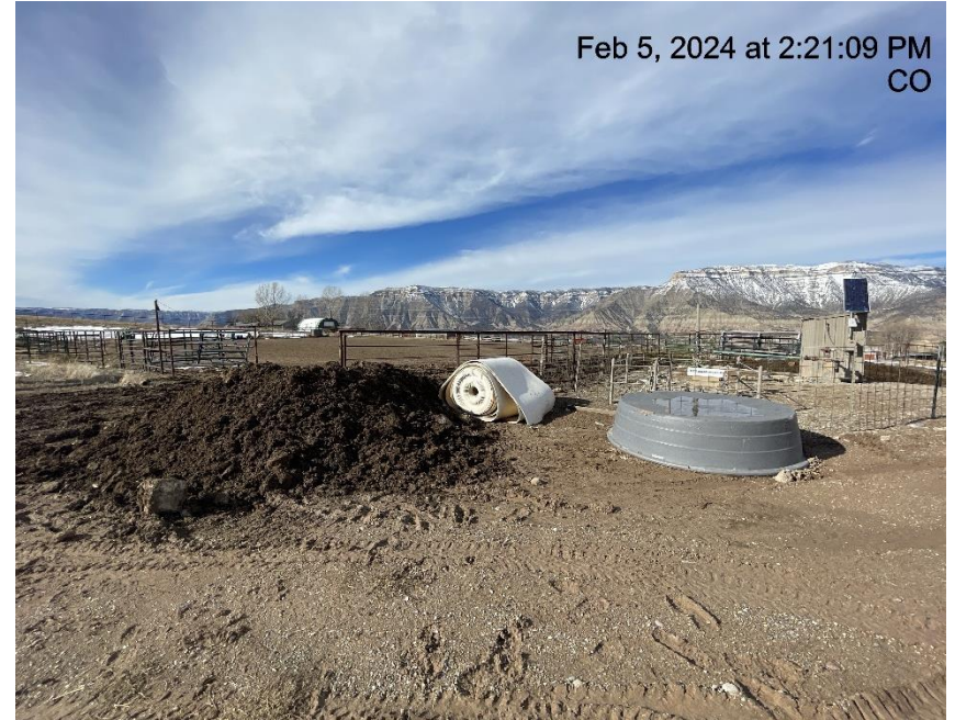
Photo # 5829 Stockpiled soils with no BMP's & debris
