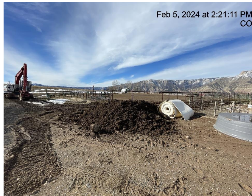
Photo # 5831 Stockpiled soils on location with no BMP's
