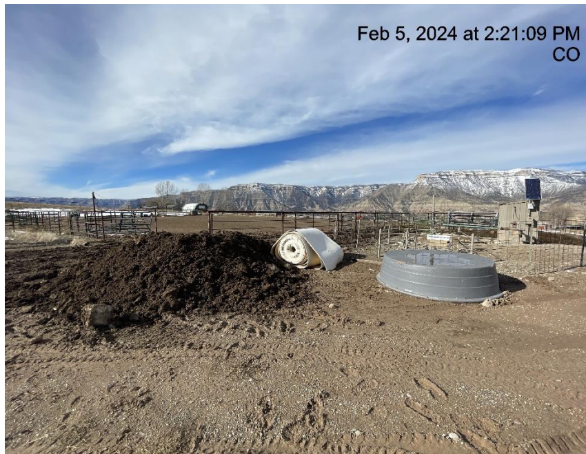
Photo # 5830 Stockpiled soils on location with no BMP's
