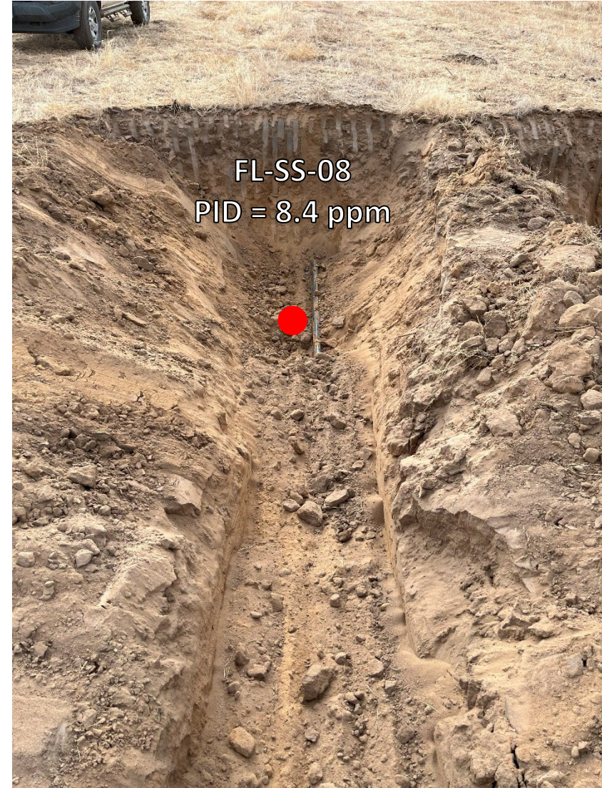
Looking southwest at bellhole/change in direction
