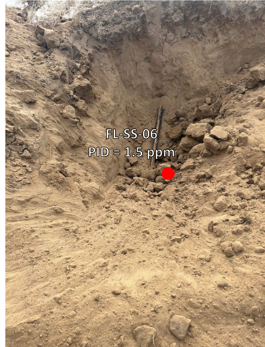
Looking south at bellhole/change of direction
