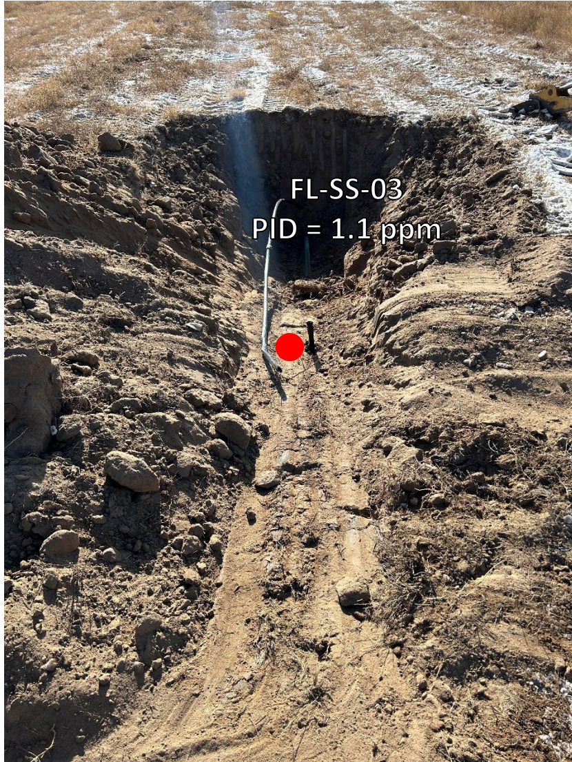
Looking southwest at bellhole/change in direction
