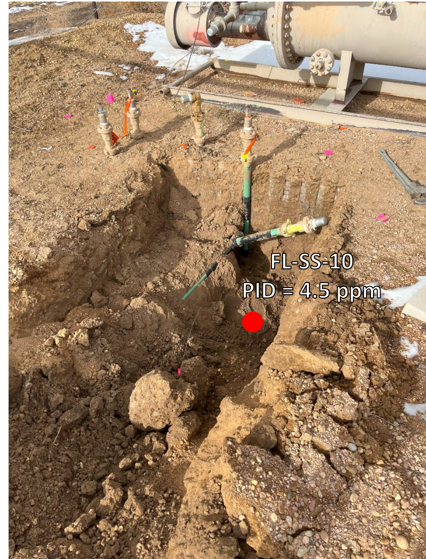
Looking north at Pt. B/terminus at separator
