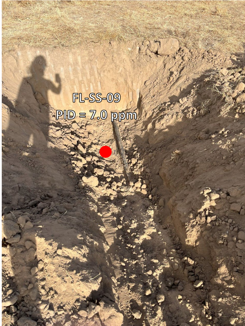
Looking northeast at bellhole/cut point for removal
