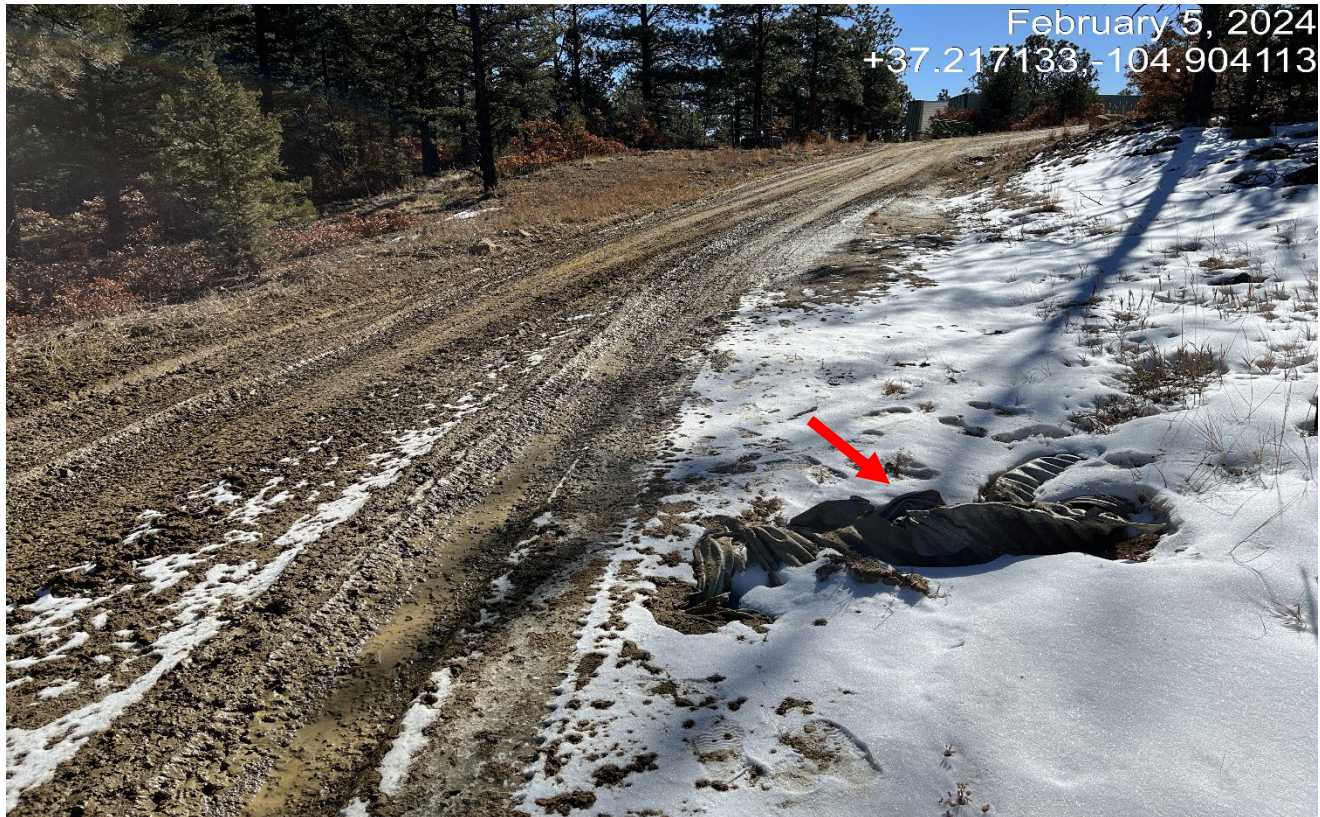
Photo 1. Facing southeast along the access road. This culvert near the wellsite is damaged and needs to be replaced.
