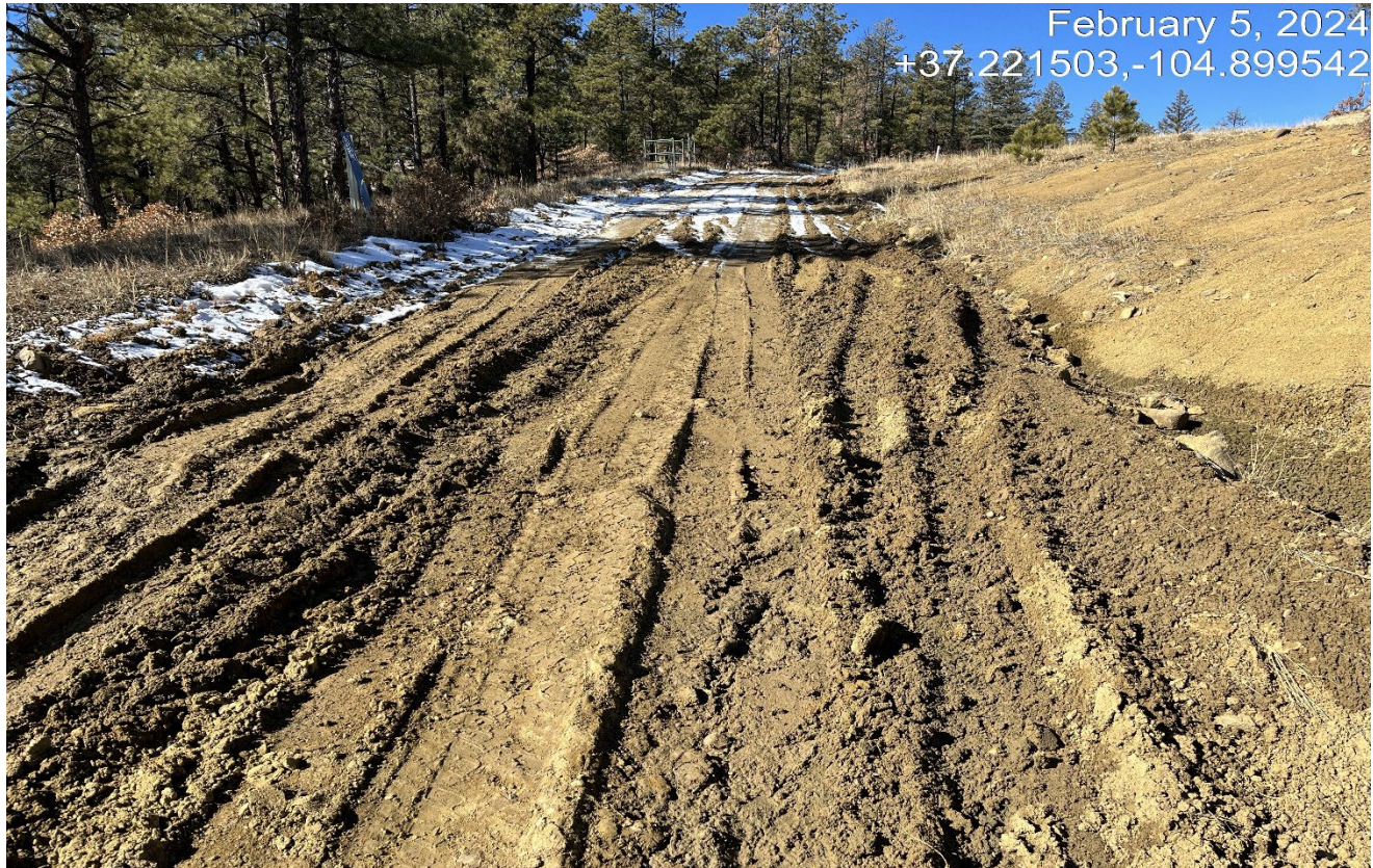
Photo 2. Facing west along the access road which is rutted and not maintained.
