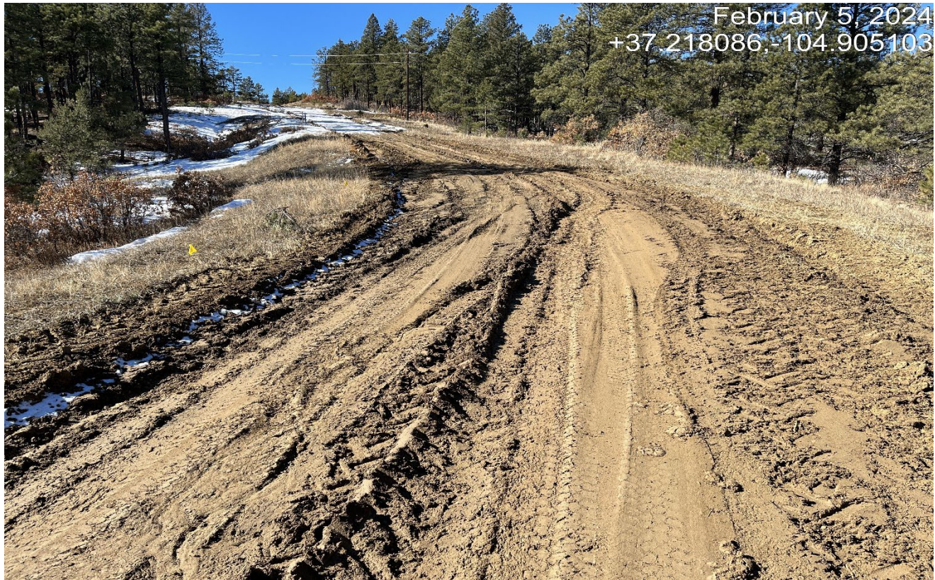
Photo 1. Facing west along the access road which is rutted and not maintained.
