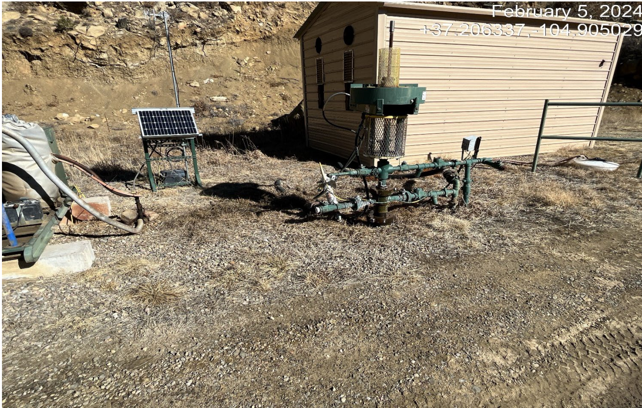
Photo 2. Facing toward the wellhead. There is a dripping leak that needs to be repaired.
