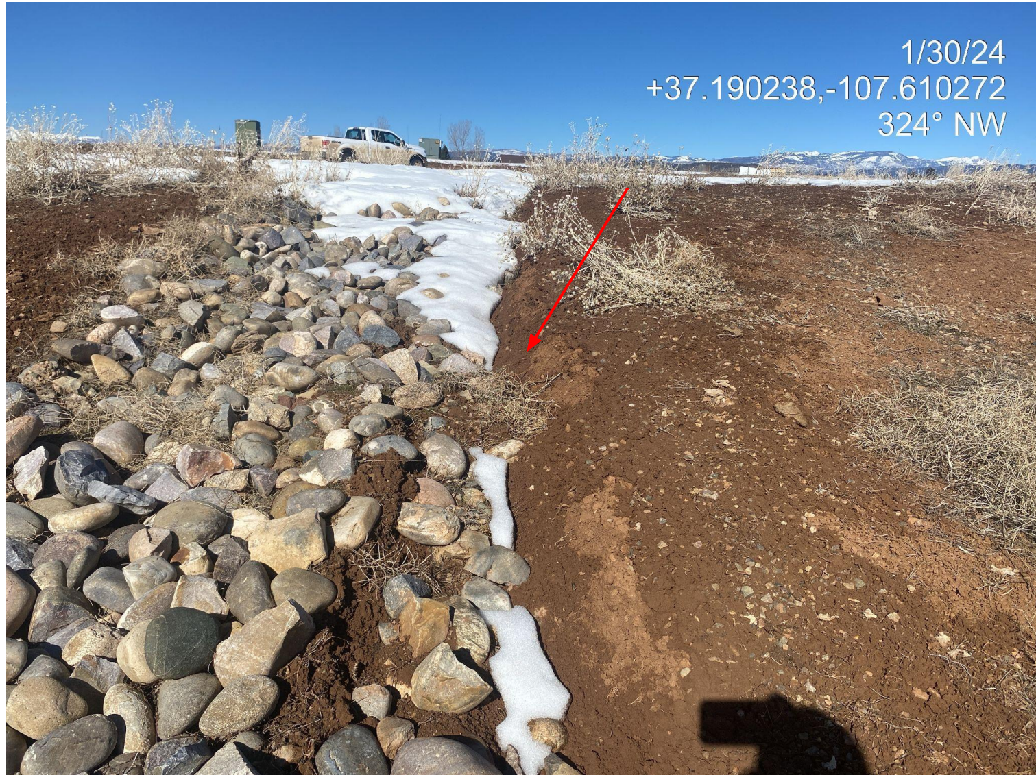
Photo 3. View of erosion forming along installed stormwater BMPs. Current stormwater round river rock BMPs remain inadequate for this area.
