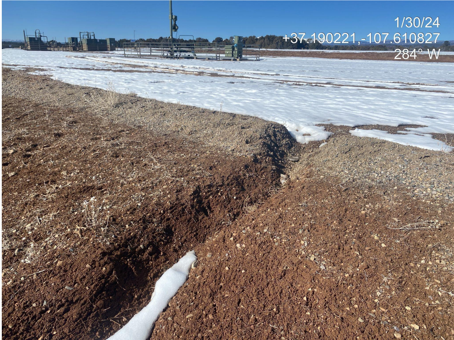
Photo 4. Additional gully erosion observed forming in the southern interim reclamation area.
