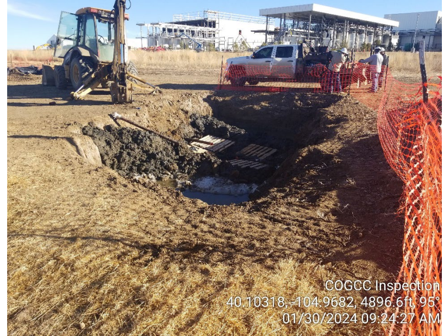
Photo 32 - Open excavation 1/30/2024 AM. Flowline repair in progress.
