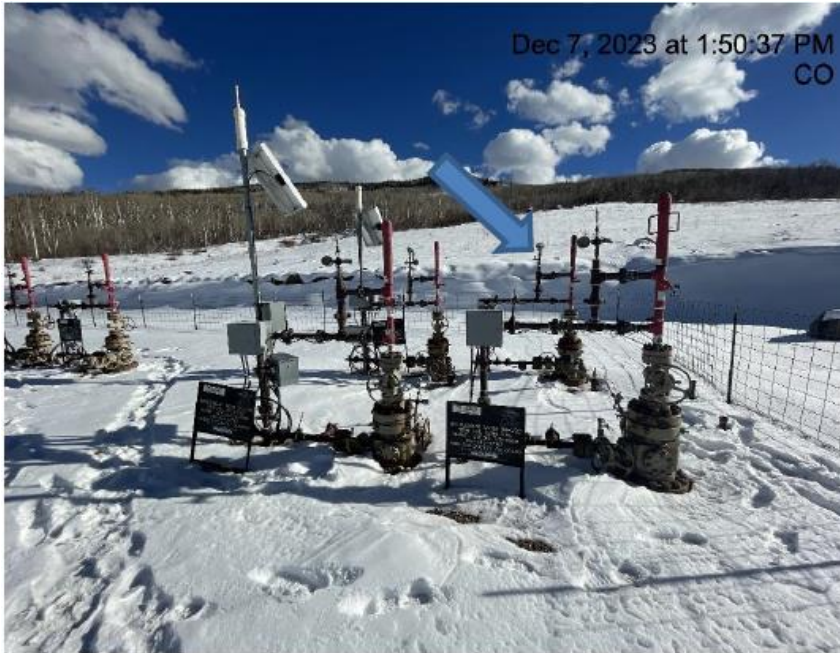
Photo # 8924 From inspection 708902473 conducted on 12/07/2023 Wellhead lacks required signage
