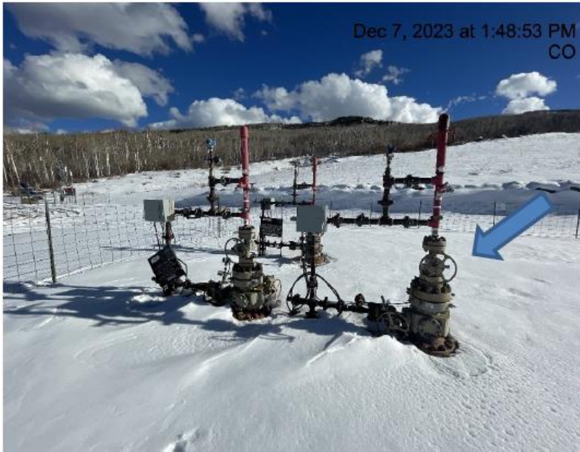
Photo # 8923 From inspection 708902473 conducted on 12/07/2023 Wellhead lacks required signage
