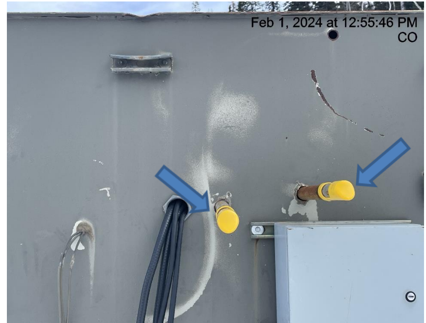
Photo # 5215 PRV & rupture disc vent lines terminate in an unsafe manner
