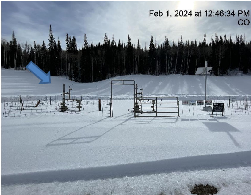
Photo # 5212 Wellhead lacks required signage
