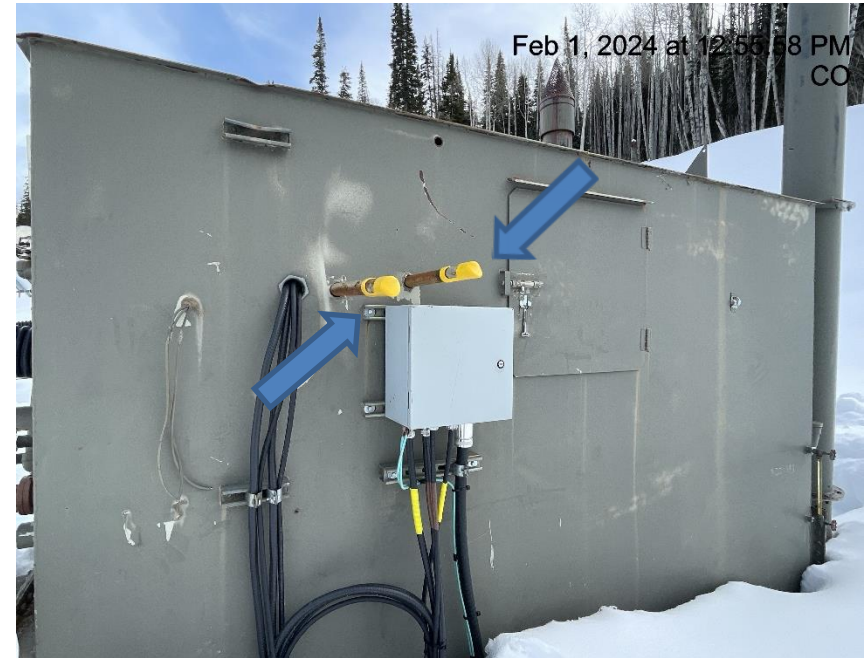
Photo # 5214 PRV & rupture disc vent lines terminate in an unsafe manner
