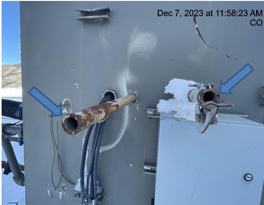
Photo # 8784 From inspection 708902455 conducted on 12/07/2023 PRV & rupture disc vent lines terminate in an unsafe manner
