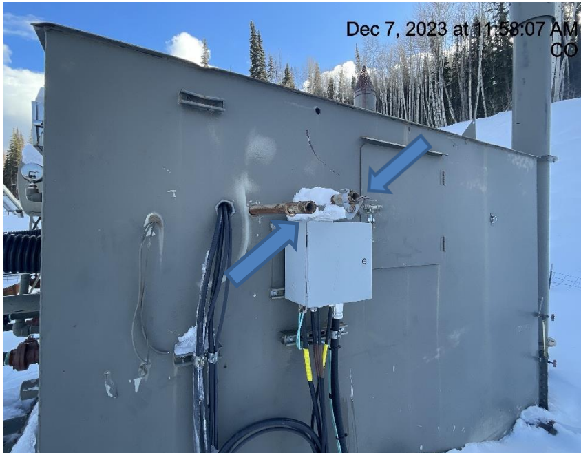
Photo # 8783 From inspection 708902455 conducted on 12/07/2023 PRV & rupture disc vent lines terminate in an unsafe manner
