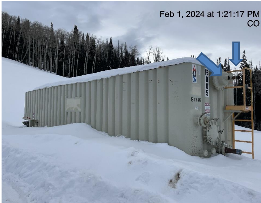
Photo # 5259 Open ended piping/wildlife hazards/available for entry by wildlife
