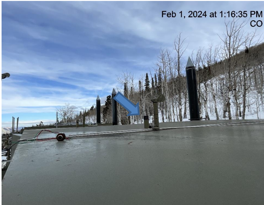
Photo # 5257 Rupture disc vent line lacks cap
