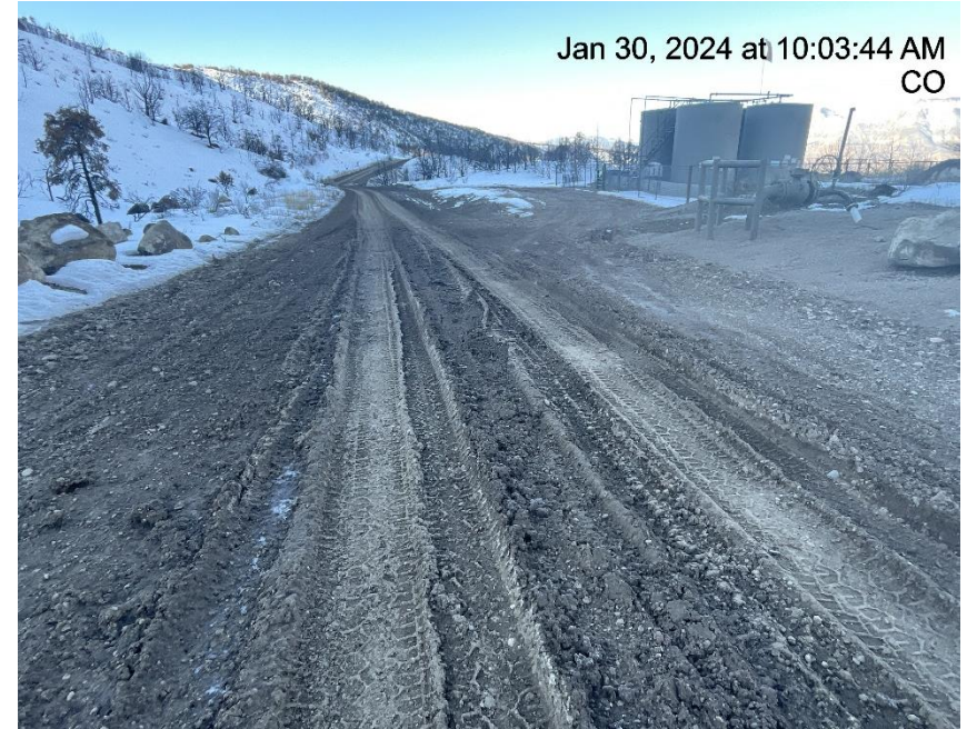
Photo # 4665 Lack of stabilization/compaction
