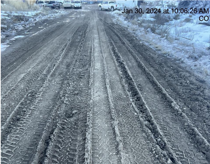
Photo # 4664 Lack of stabilization/compaction
