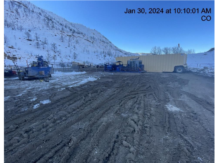
Photo # 4669 Lack of stabilization/compaction
