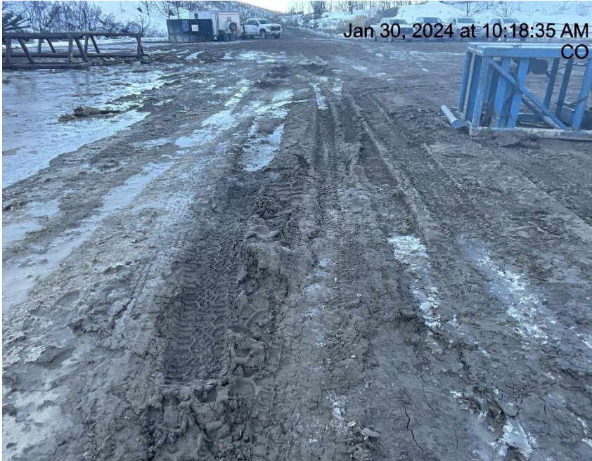
Photo # 4676 Lack of stabilization/compaction
