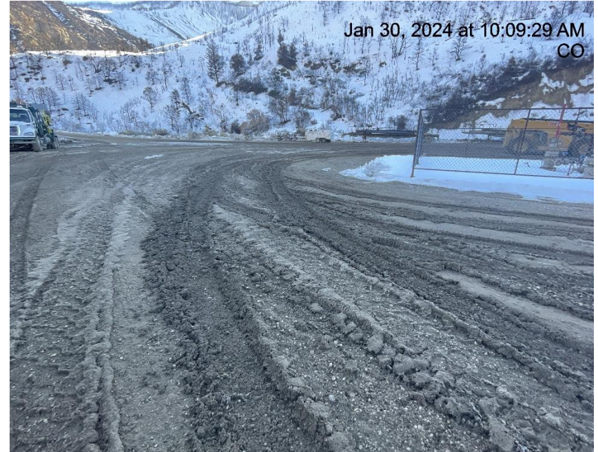
Photo # 4667 Lack of stabilization/compaction
