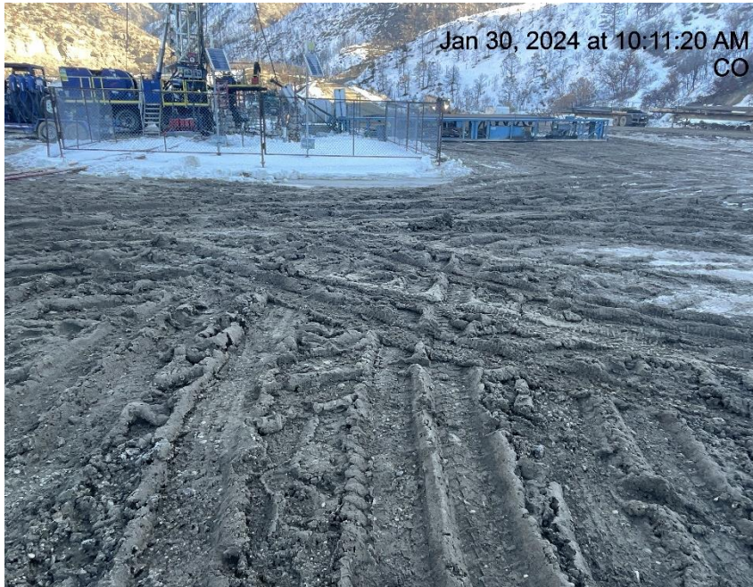
Photo # 4670 Lack of stabilization/compaction
