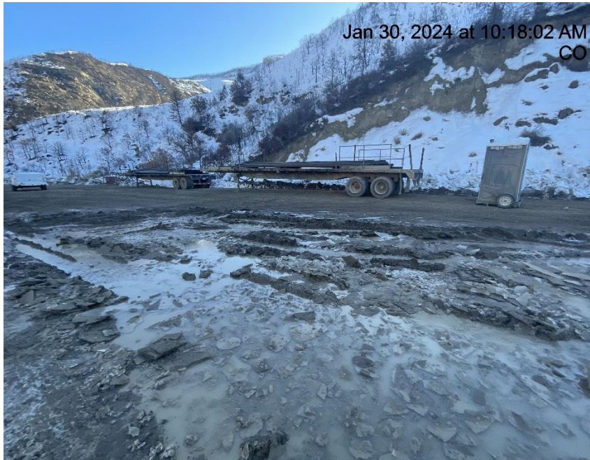
Photo # 4672 Lack of stabilization/compaction
