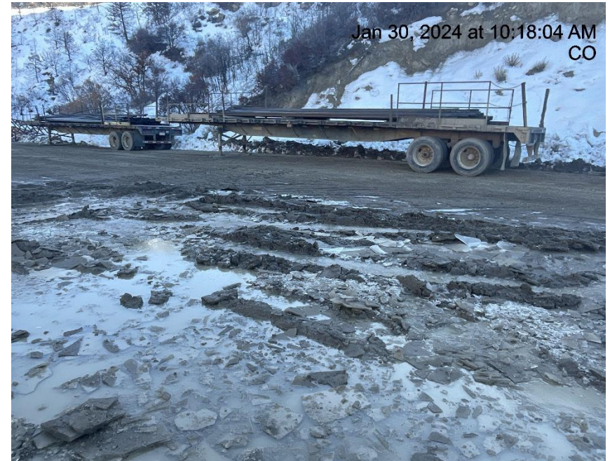
Photo # 4673 Lack of stabilization/compaction
