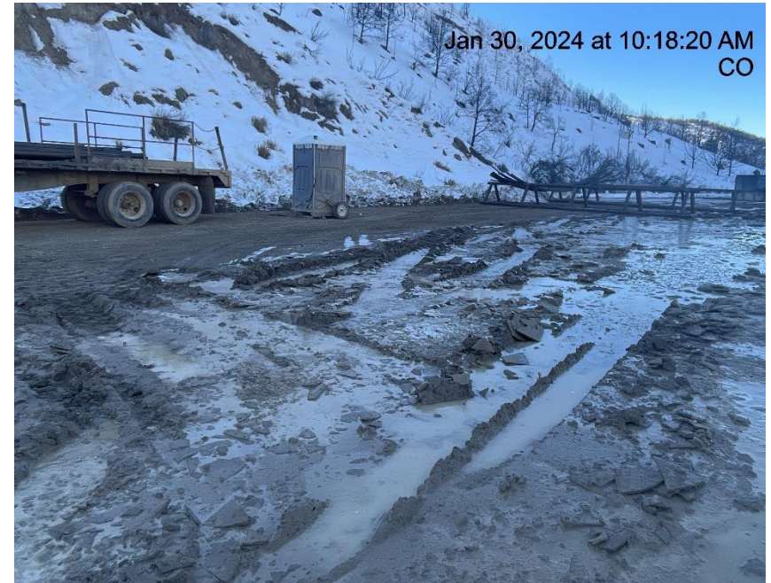
Photo # 4675 Lack of stabilization/compaction
