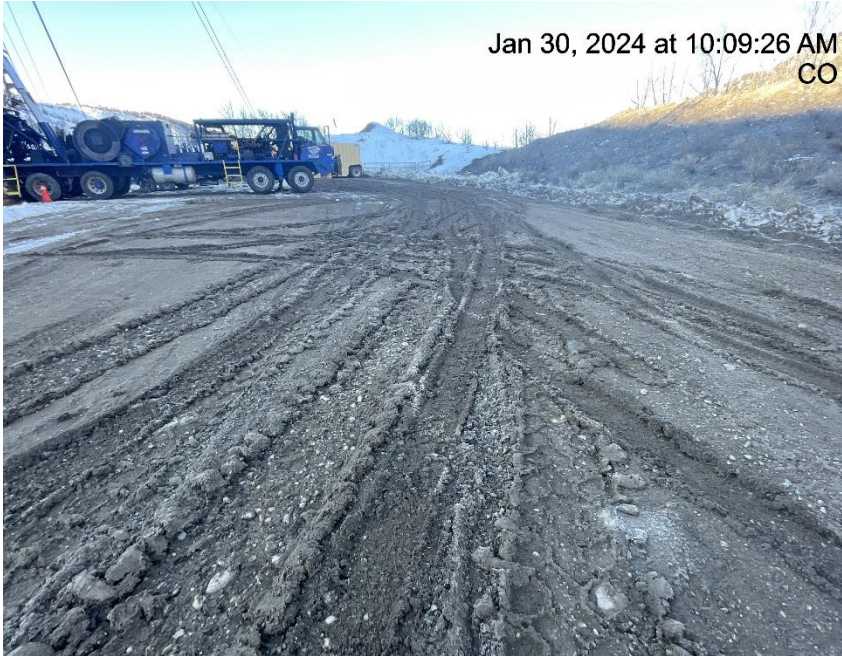
Photo # 4666 Lack of stabilization/compaction
