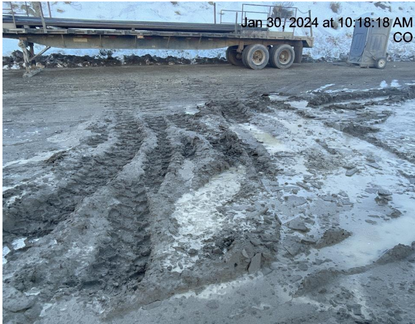
Photo # 4674 Lack of stabilization/compaction
