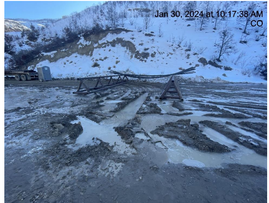
Photo # 4671 Lack of stabilization/compaction
