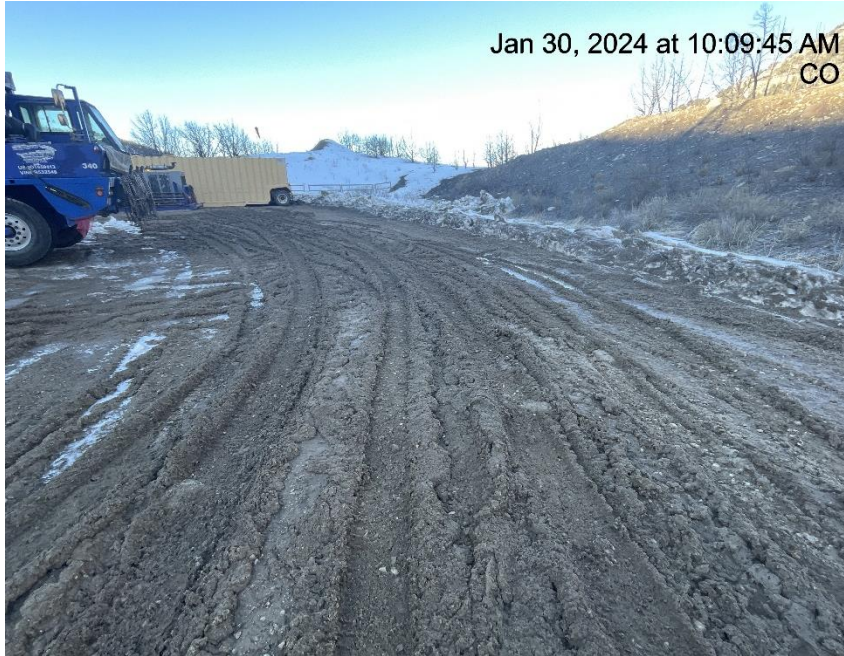
Photo # 4668 Lack of stabilization/compaction
