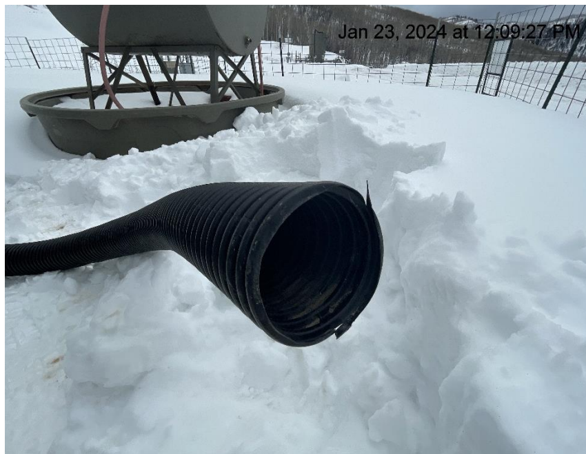
Photo # 3550 From inspection 708902863 conducted on 01/23/2024 Flowline heating insulation open ended/wildlife hazard/available for entry by wildlife
