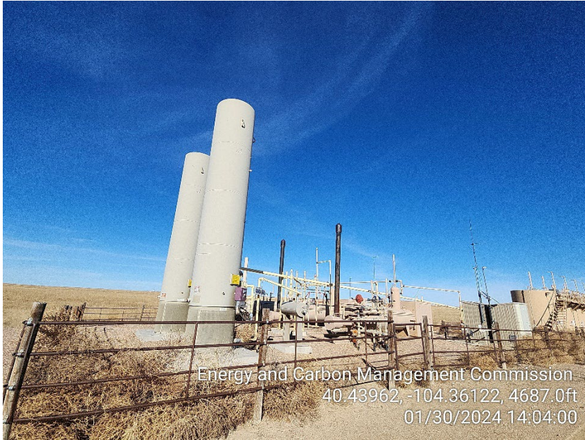
Photo 1 – ECDs and Separators
