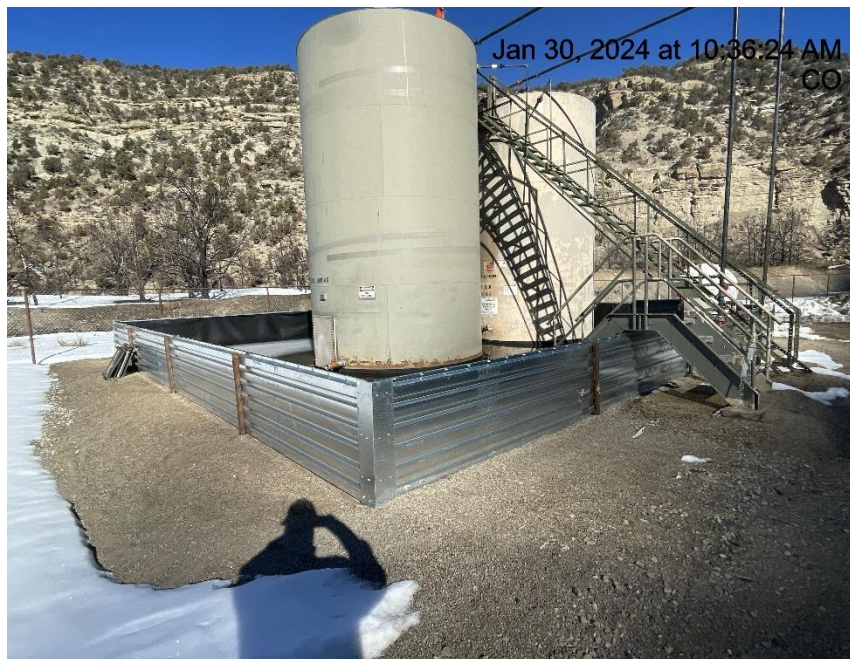
Photo # 4704 Tank battery lacks required signage
