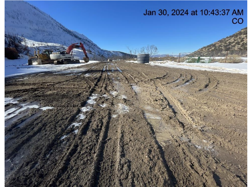
Photo # 4713 Lack of stabilization/compaction
