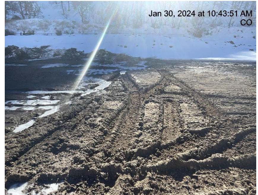
Photo # 4715 Lack of stabilization/compaction
