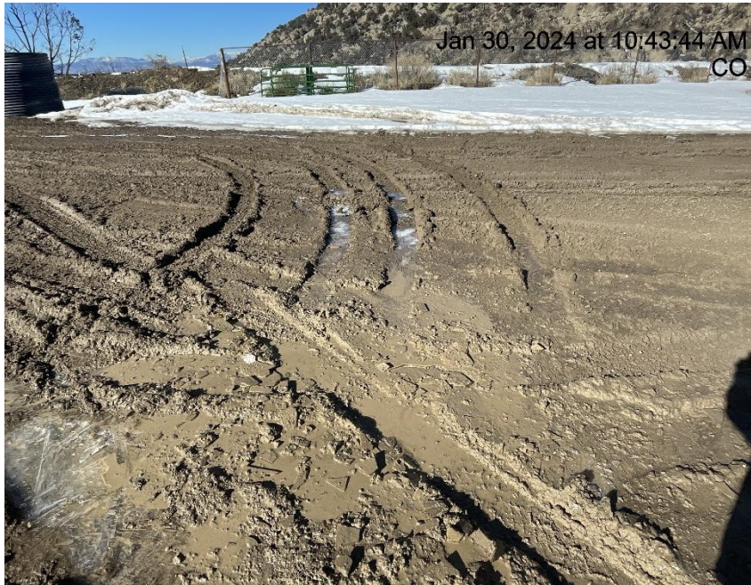
Photo # 4714 Lack of stabilization/compaction
