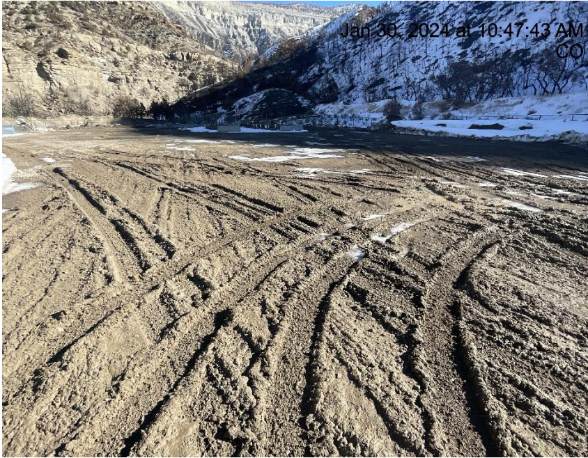
Photo # 4718 Lack of stabilization/compaction
