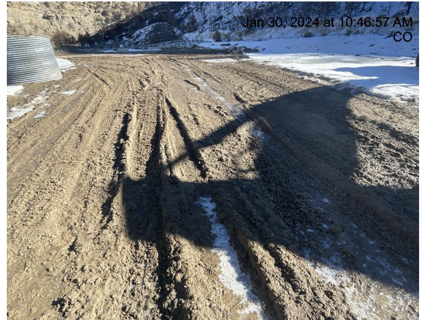
Photo # 4717 Lack of stabilization/compaction
