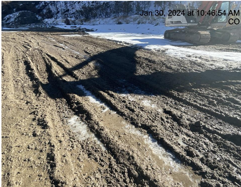
Photo # 4716 Lack of stabilization/compaction
