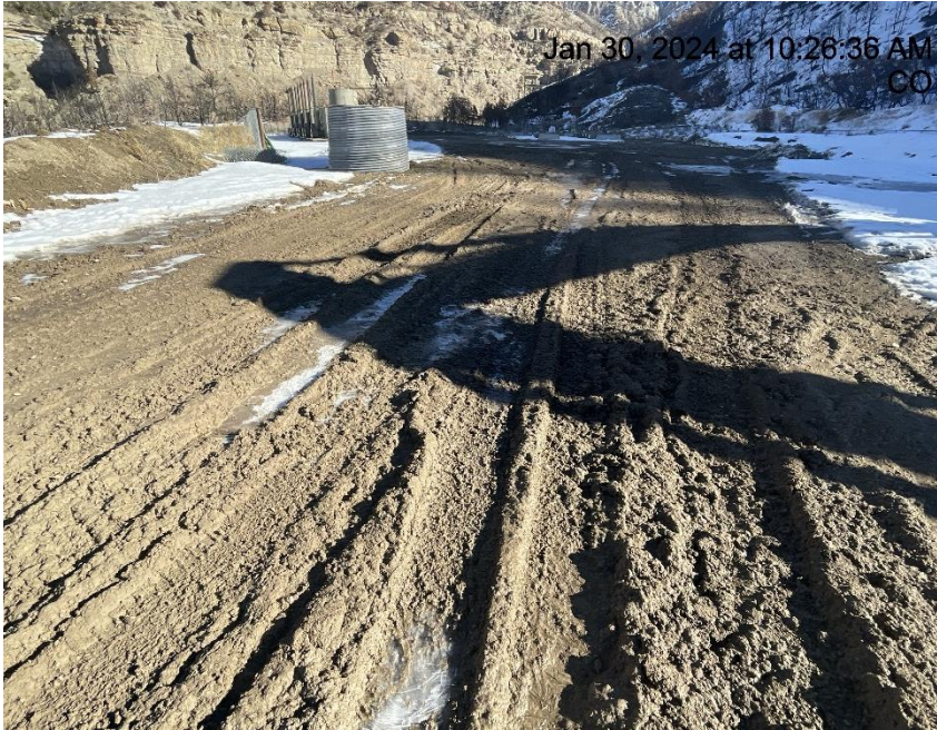
Photo # 4712 Lack of stabilization/compaction
