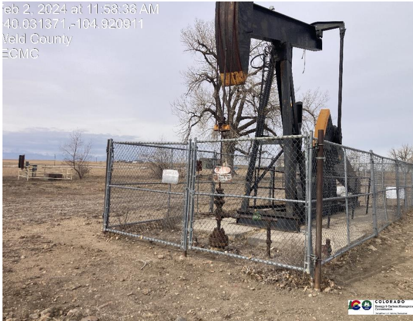
Pic 1 wellhead / pumpjack
