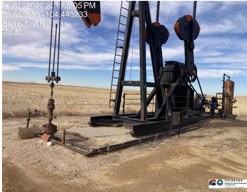
Pic 1 Wellhead / pumpjack
