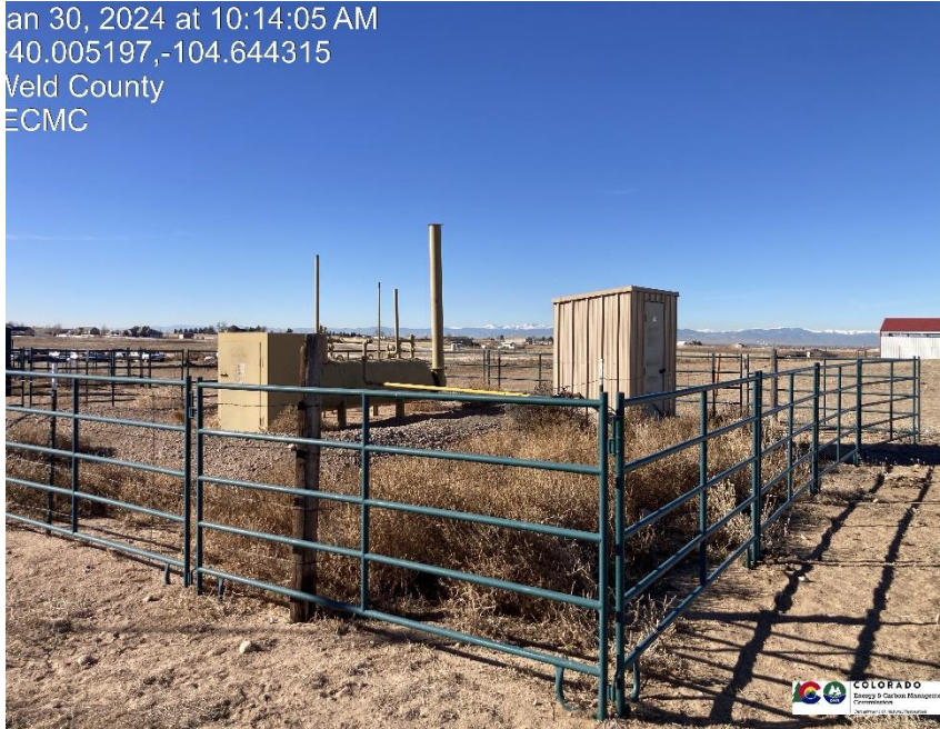
Pic 3 separator, GMR, weeds unmanaged
