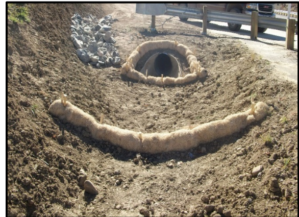
Erosion Logs along construction access road
