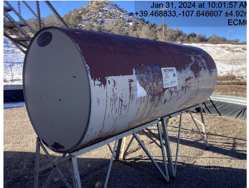
Methanol tank lacking operator info
