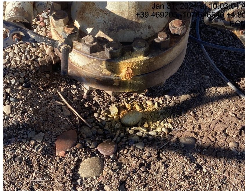
Well head leaking
