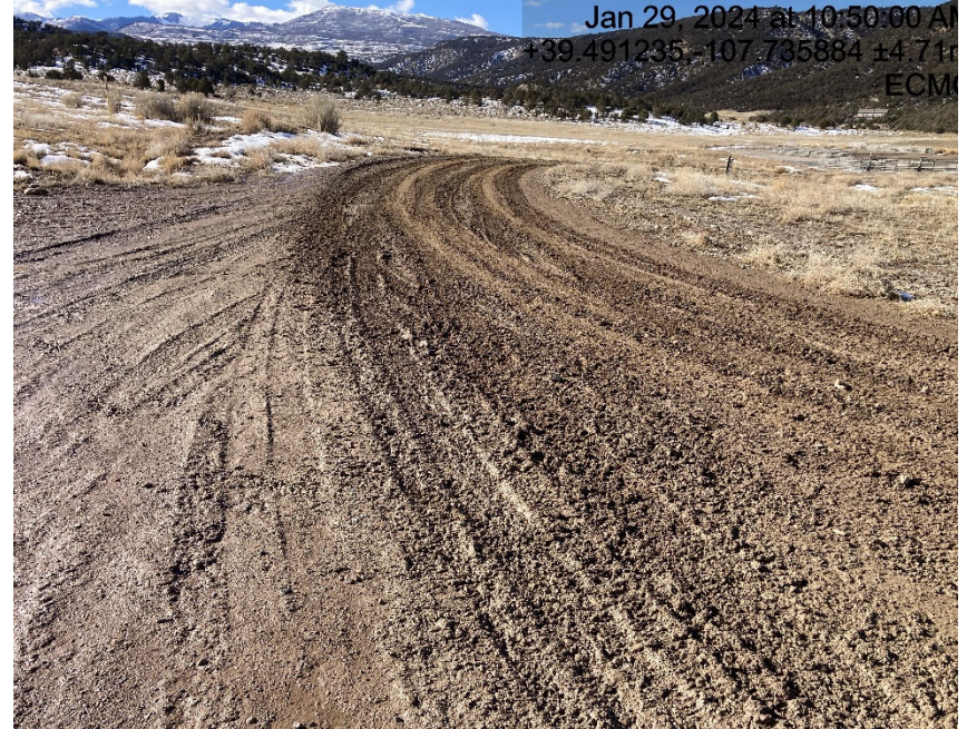
Location entrance shows lack of stabilization and tracking
