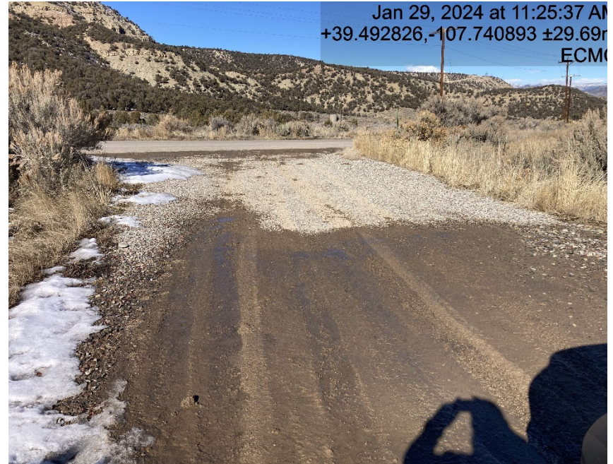
Access road entrance tacking BMP's need maintained
