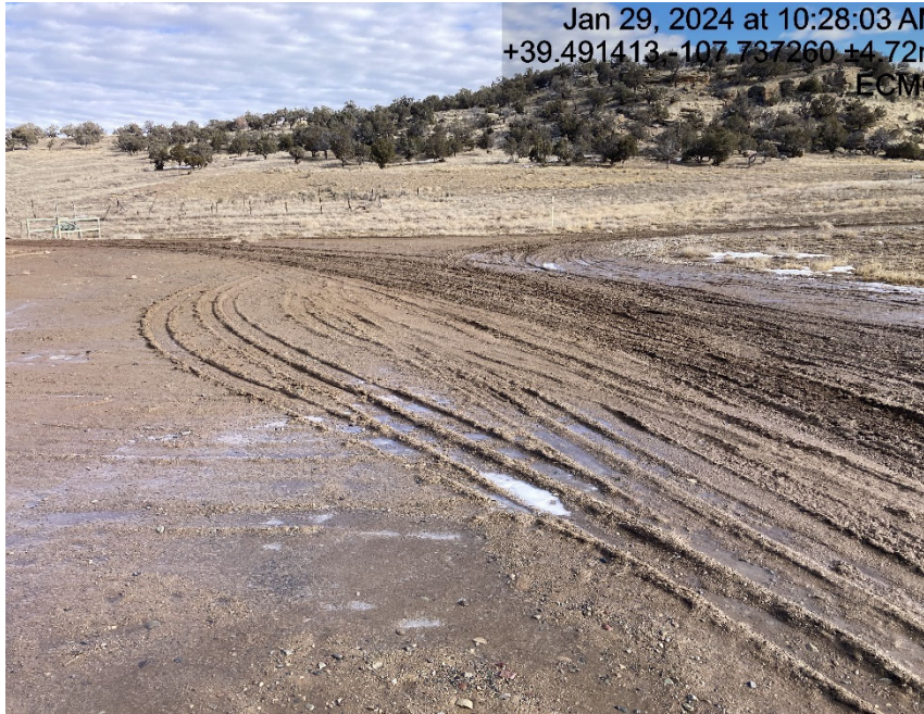
Location entrance shows lack of stabilization
