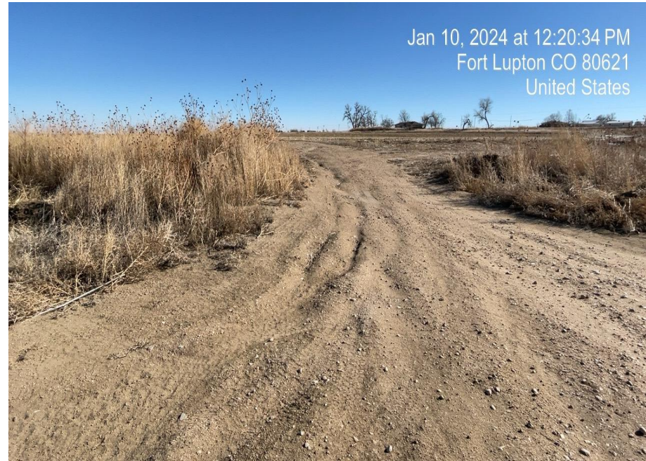
Photo 6. Photo taken of access road stormwater erosion. . Photo taken facing northwest.
