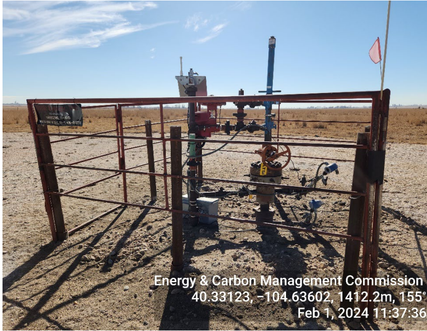
Photo 3: SI Wellhead
