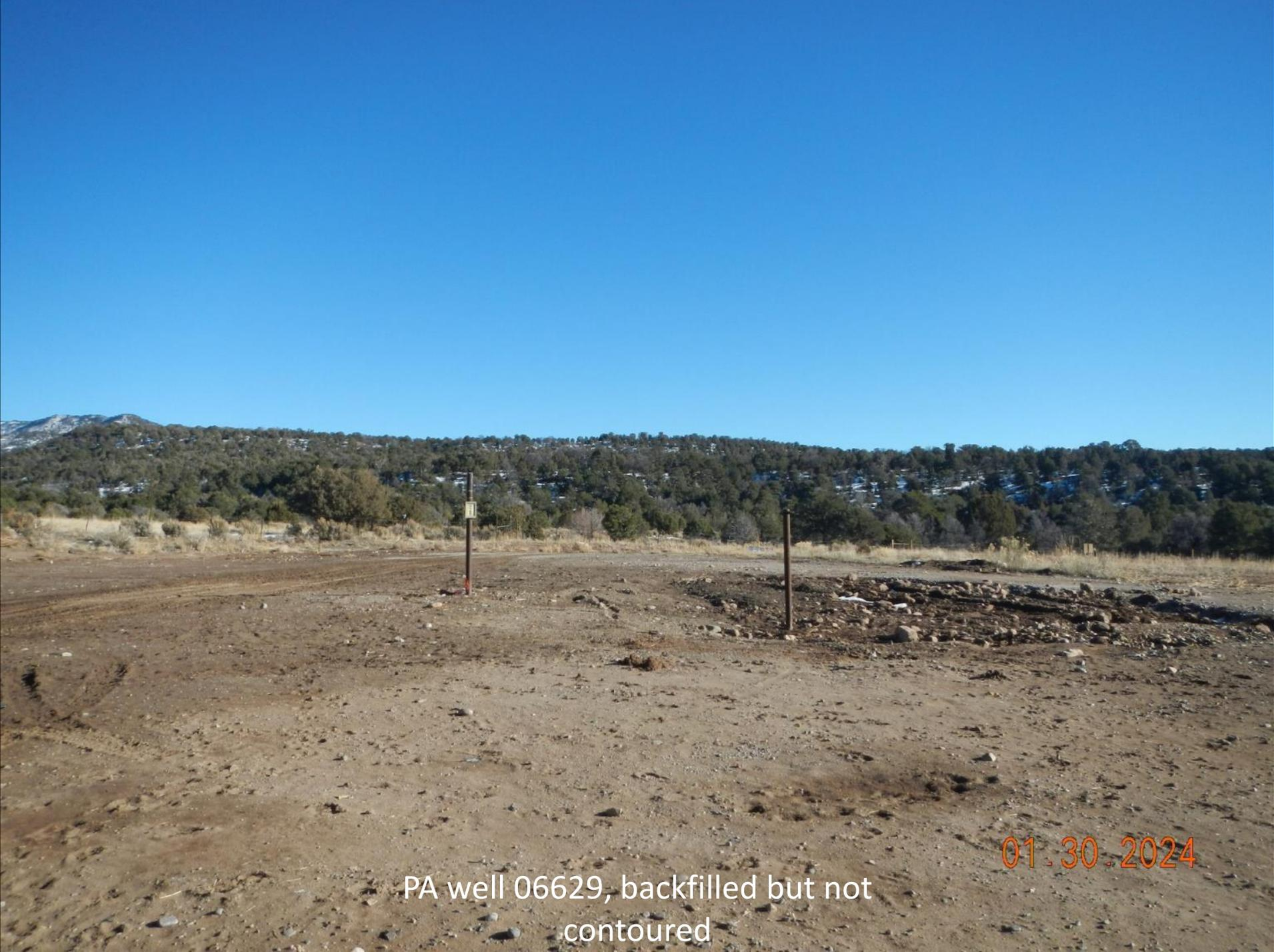
PA well 06629, backfilled but not
