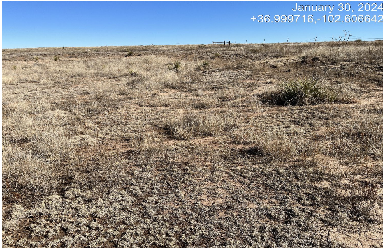
Photo 5. Facing east toward the location cut slope. The cut slope needs to be recontoured with fill slope material to match pre-existing grade..
