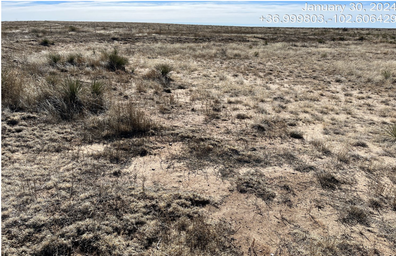
Photo 4. Facing southwest toward the location cut slope. The cut slope needs to be recontoured with fill slope material to match pre-existing grade.
