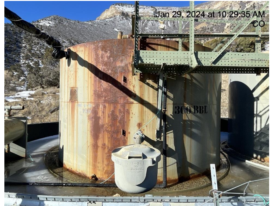
Photo # 4375 Production tank lacks required labeling
