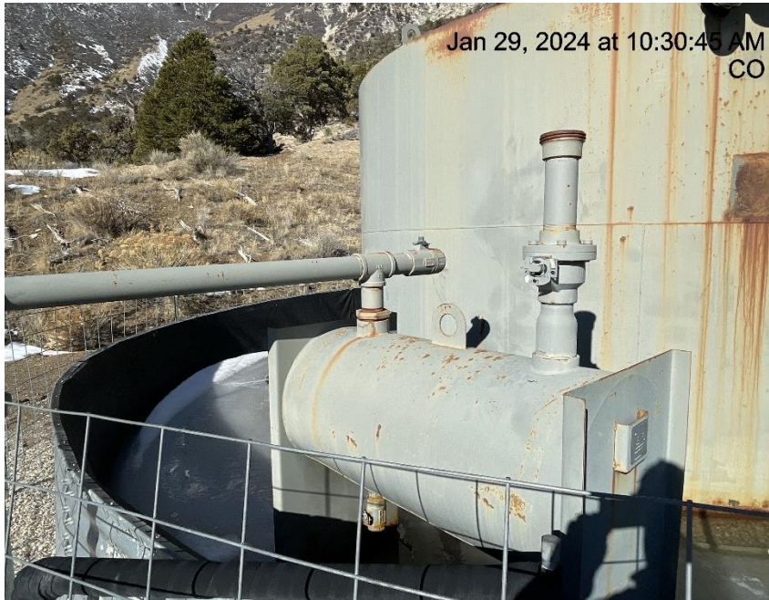
Photo # 4372 Knock out drum for ECD disconnected from tanks
