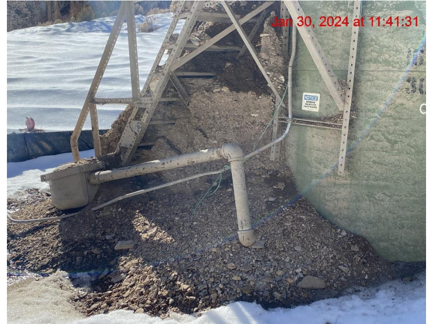
Tank Overrun by Sediment – Photo #08908
