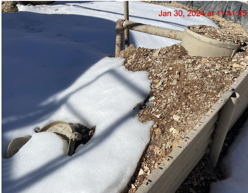
Secondary Containment/Production Equipment Overrun by Sediment – Photo #08909
