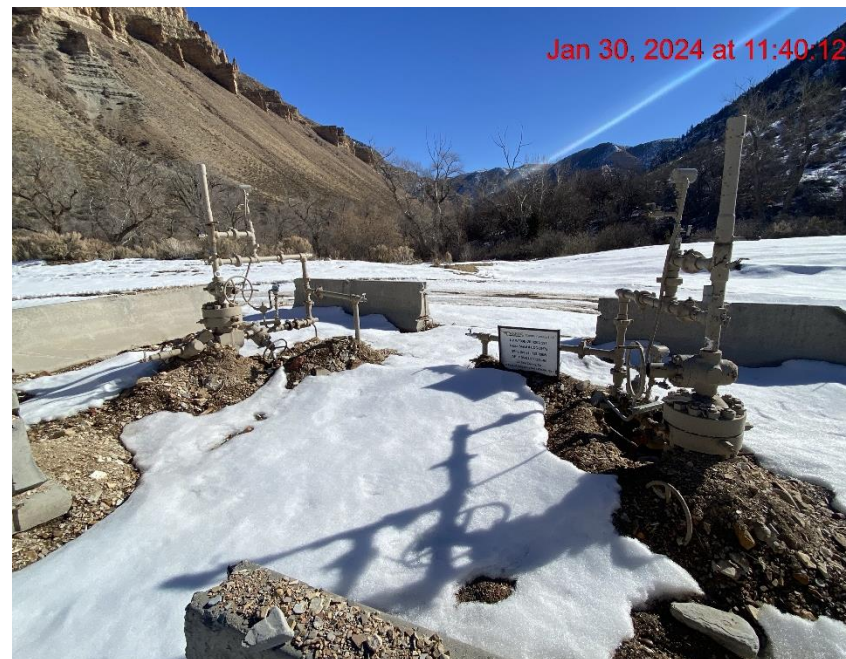
Wellheads/Sediment Encroachment – Photo #08903
