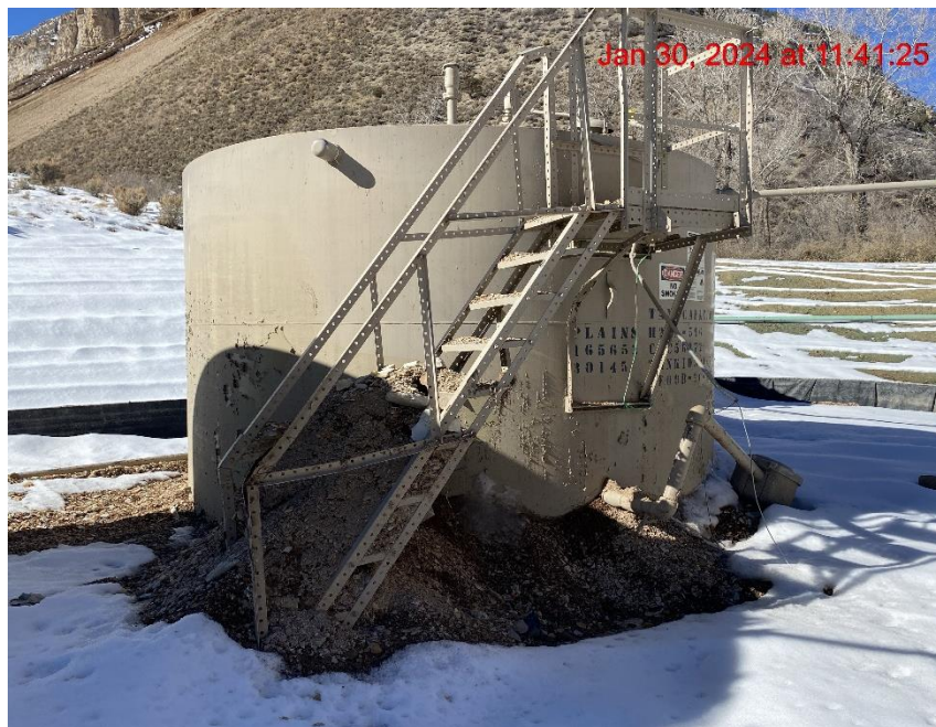
Tank Overrun by Sediment – Photo #08907
