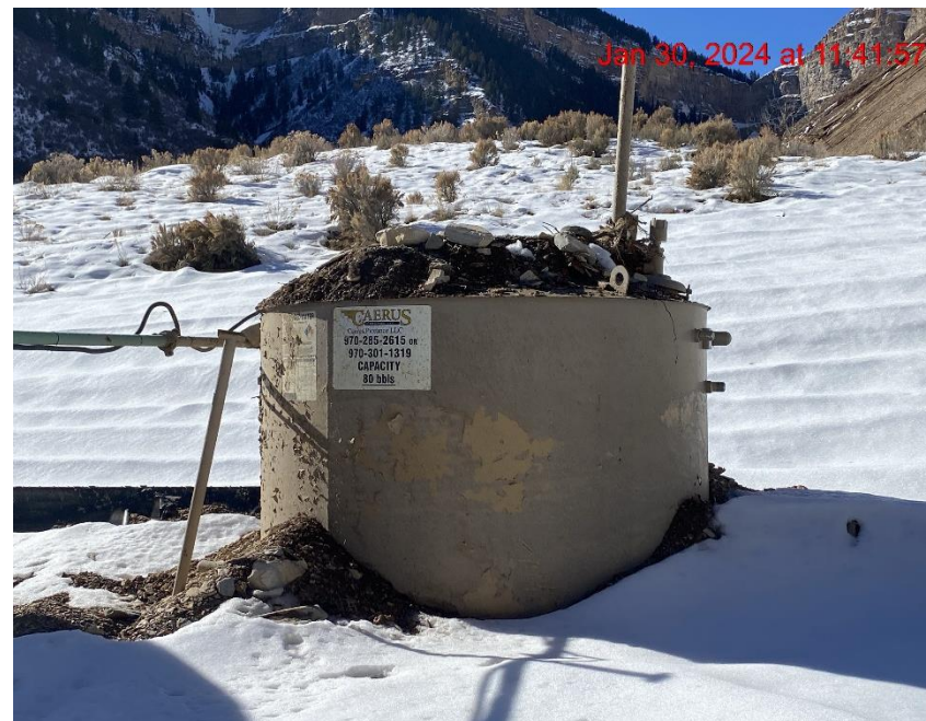
Tank Overrun by Sediment – Photo #08910
