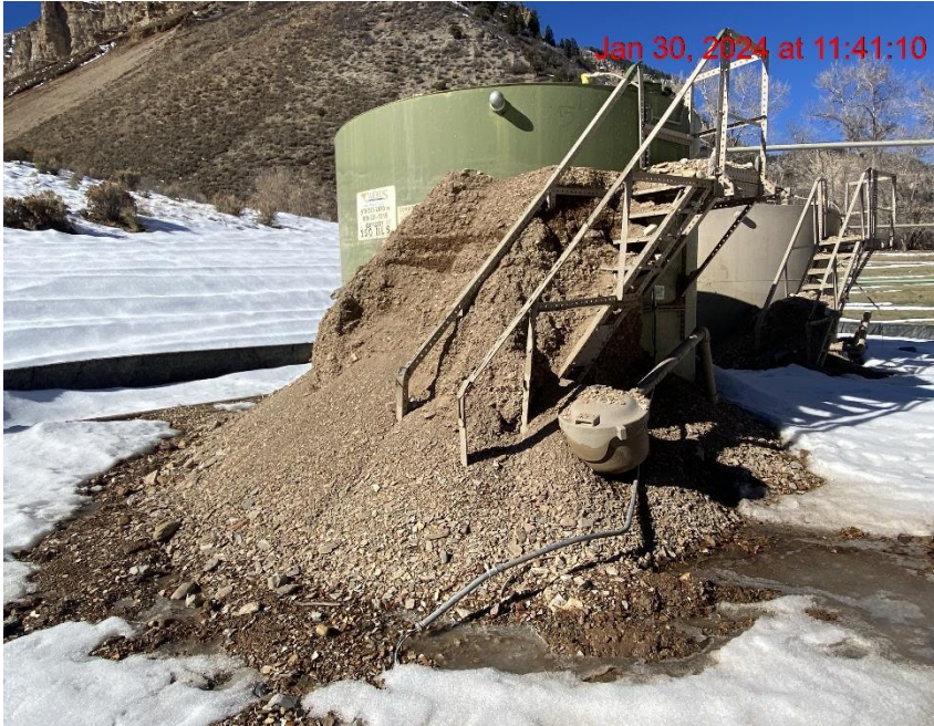
Tank Overrun by Sediment – Photo #08906
