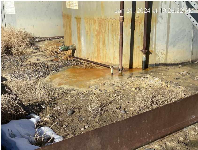
Oily waste on tank and on the ground
