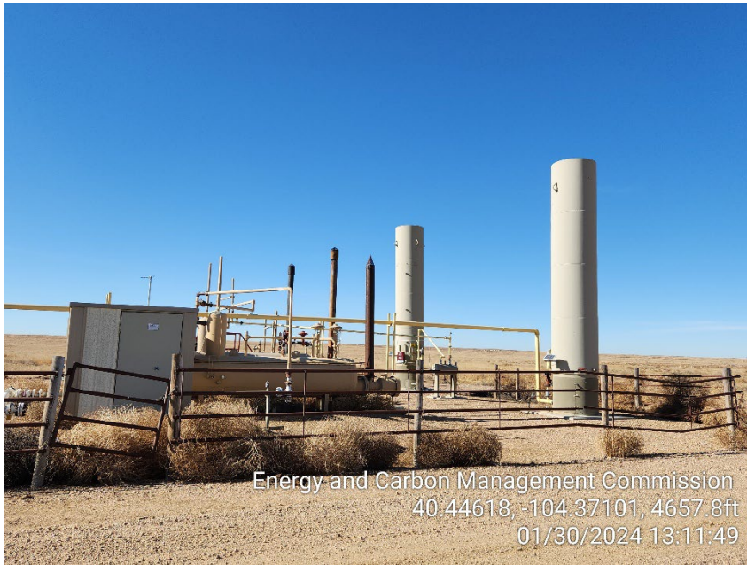
Photo 1 – Separators and ECDs
