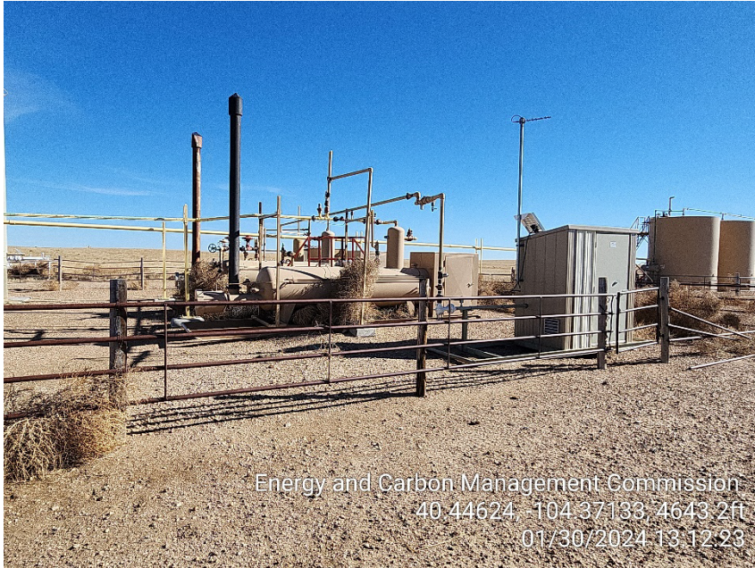
Photo 3 – Separators and Gas Meter House
